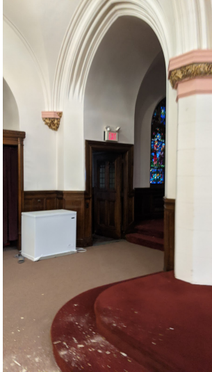
View Towards Exit Discharge #1
