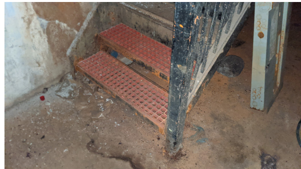
Stairs at the bottom of the Mech room
