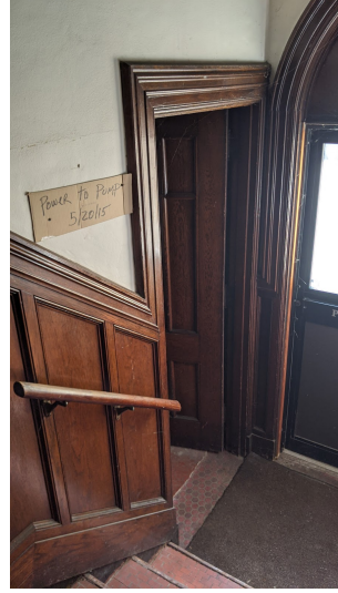
View Towards Exit Discharge #1
