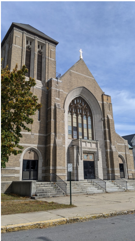
Exterior from St Mary Street
