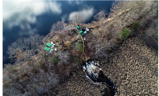
Emergency Response of Dam Breach with Bypass System in-place
