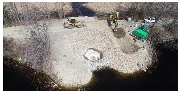
Finishing Emergency Repairs to Industries Drive Dam, Norfolk, MA
