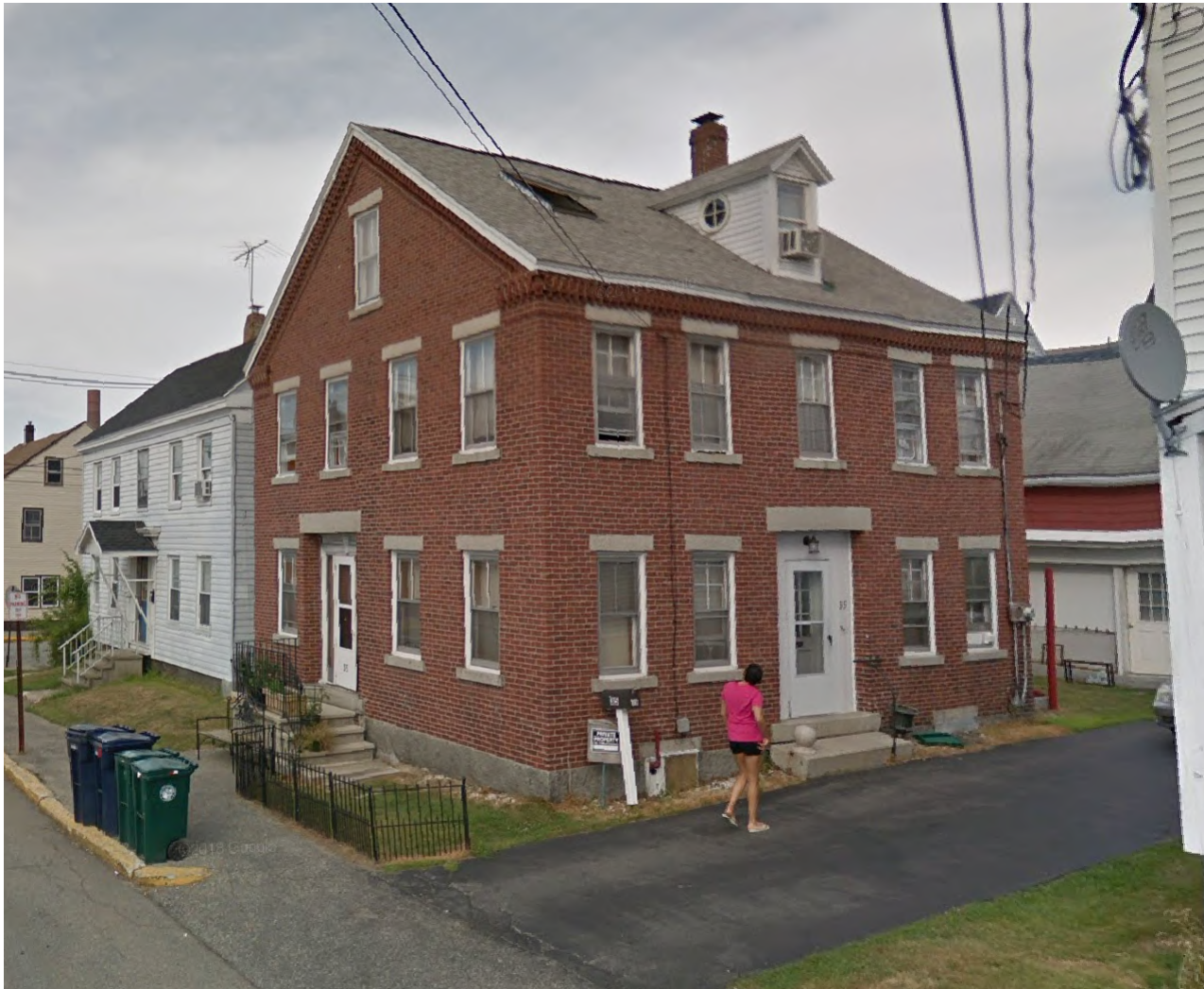
SIMILAR DORMER DESIGN ON NEIGHBORING BUILDING
