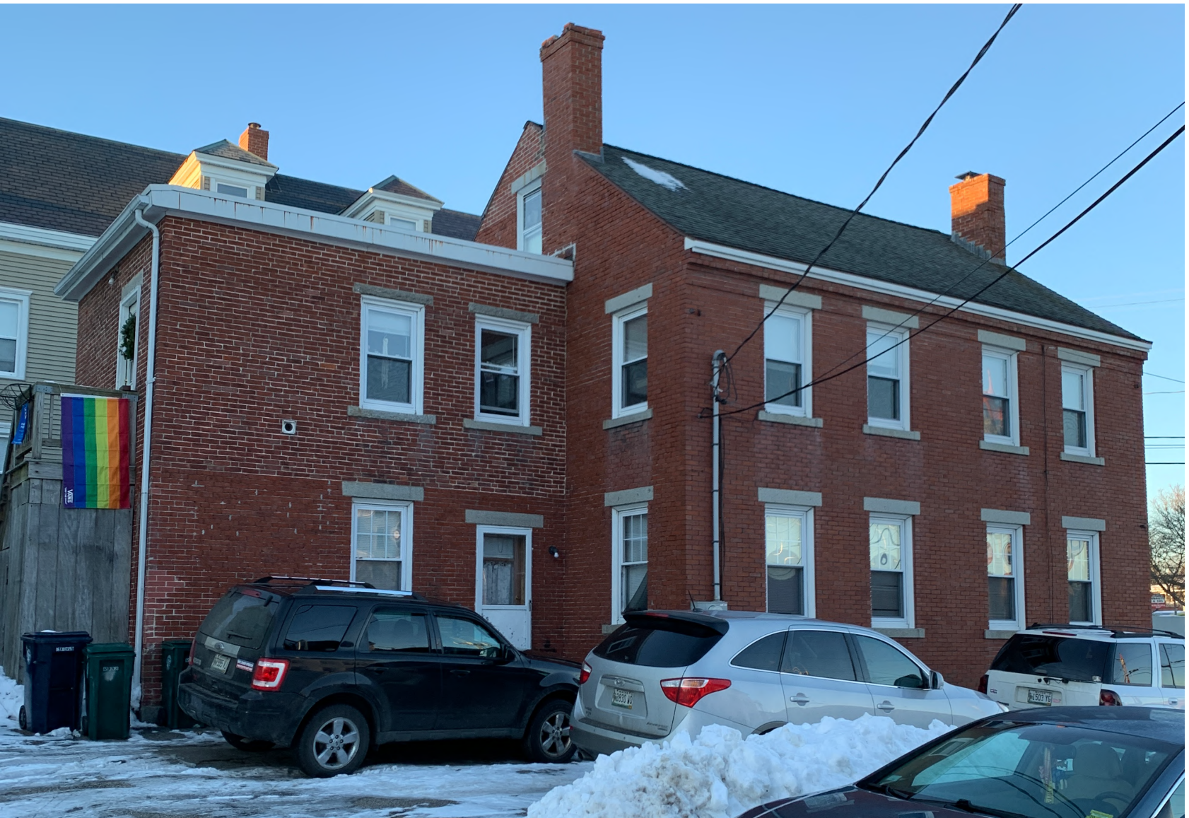
CURRENT VIEW FROM KING STREET
