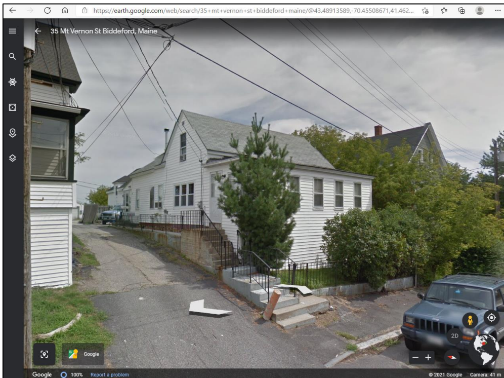
Source: "35 Mt. Vernon Street, Biddeford, Maine." 43°29'18" N 70°27'16" W. Google Earth Street View. Accessed Date: 05/03/2021.
