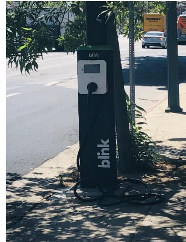
Figure 3. Sample Curbside EVCS
