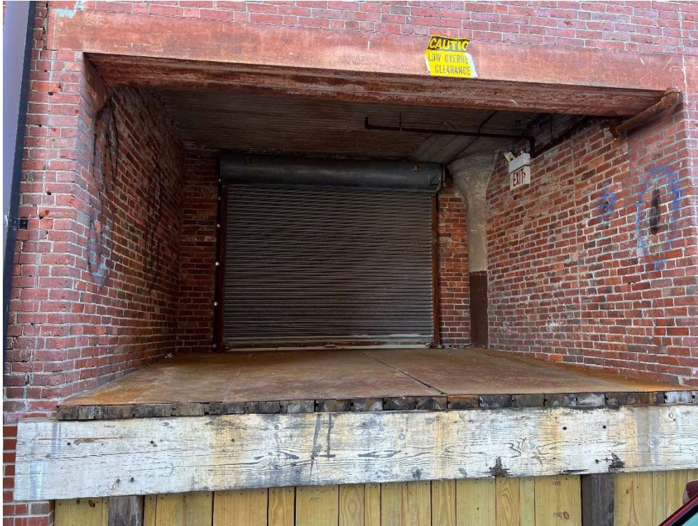
Building 36 Loading Dock (Looking South)
