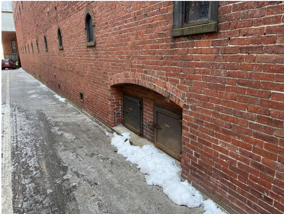
Bulkhead Doors in Rear of Existing Building (Looking Southeast)
