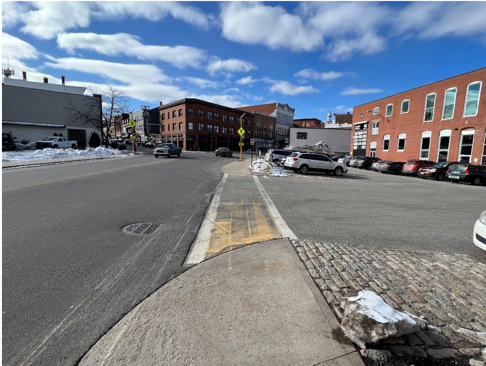
Crosswalk across Parking Lot Entrance (Looking West)
