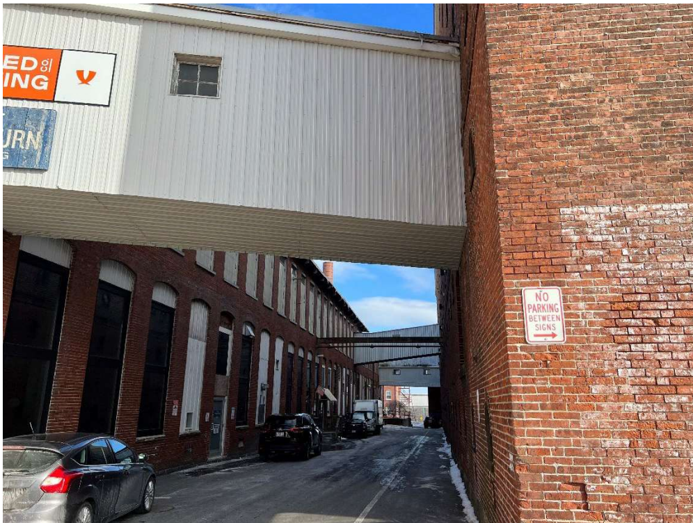
Aerial Bridge over Alleyway (Looking East)
