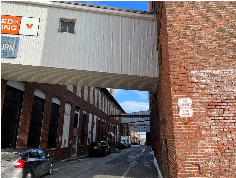
Aerial Bridge over Alleyway (Looking East)
