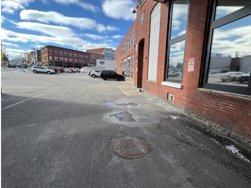
Parking Lot and 32 Main St Entrance Adjacent to Existing Building (Looking West)
