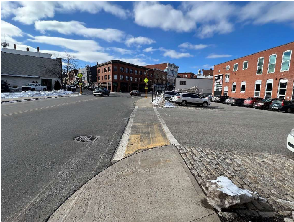
Crosswalk across Parking Lot Entrance (Looking West)
