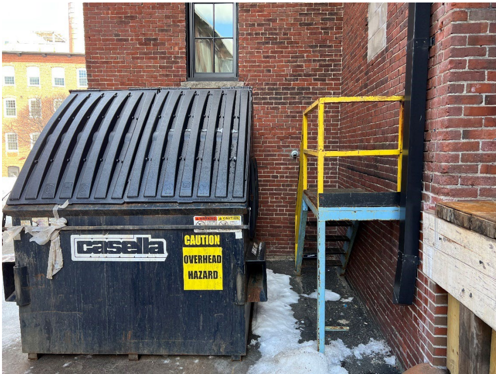
Dumpster adjacent to Building 36 Loading Dock (Looking East)
