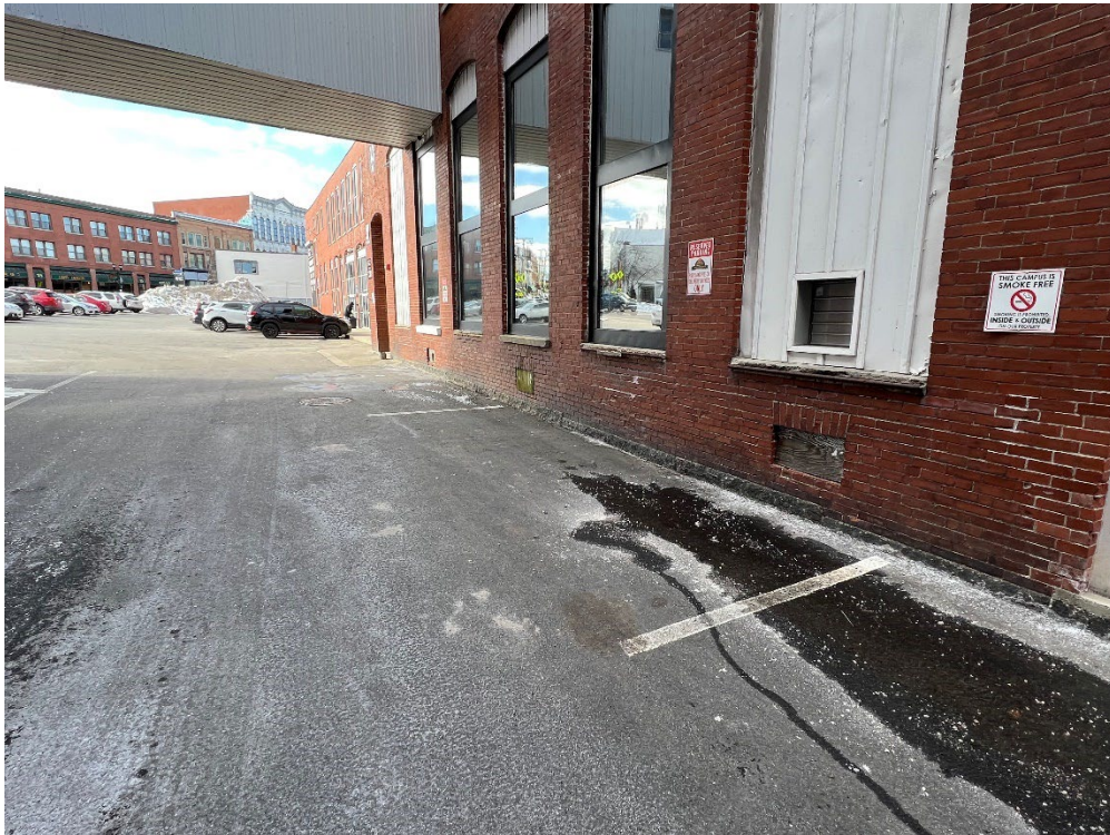
Parking Stalls Along Building 13 Building (Looking Northwest)
