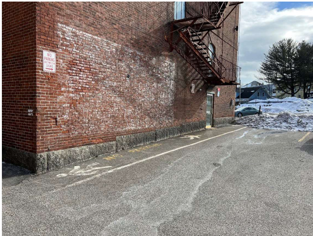
West Face of Building 36 (Looking Southeast)
