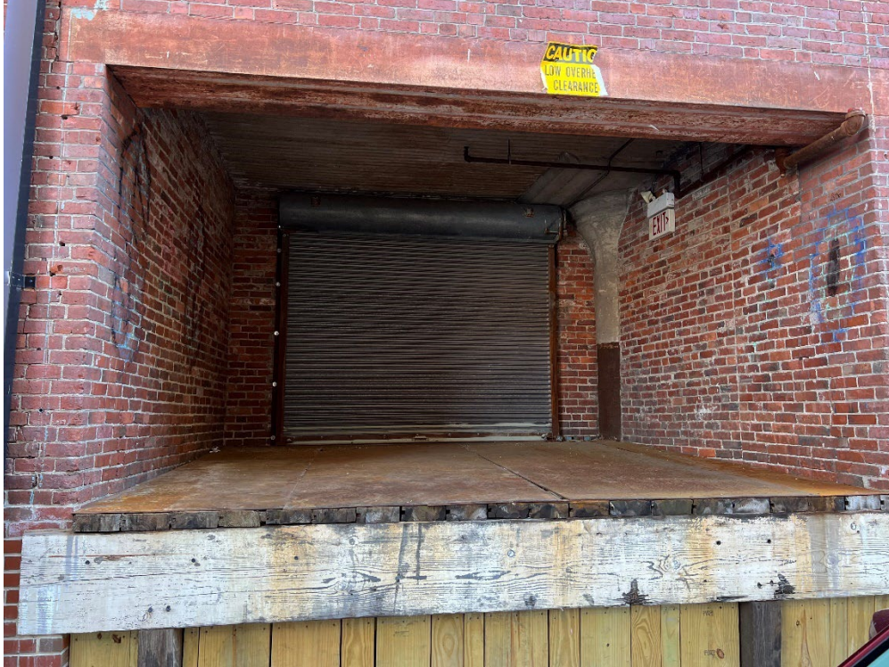
Building 36 Loading Dock (Looking South)
