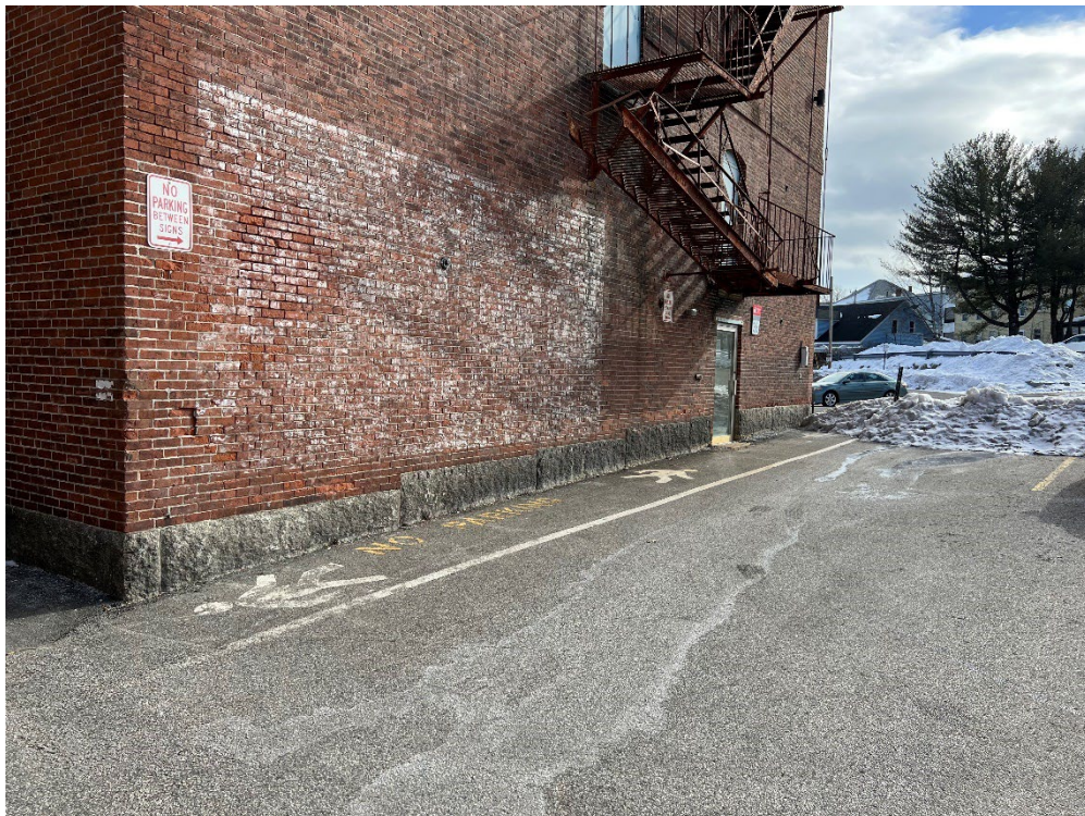
West Face of Building 36 (Looking Southeast)
