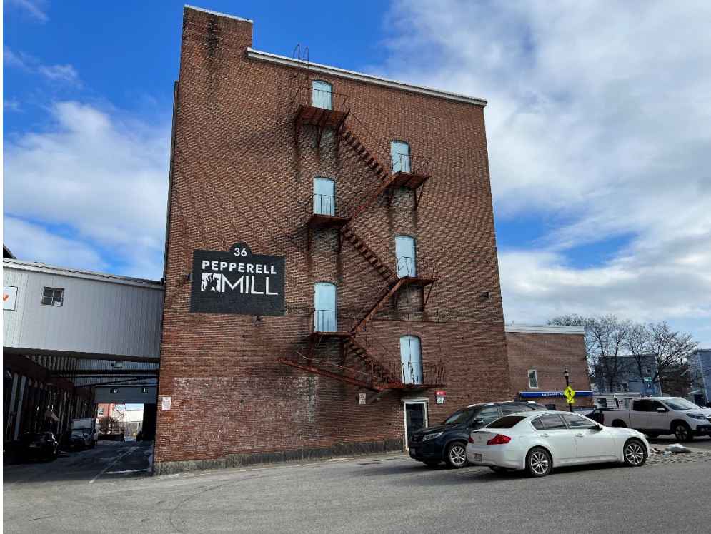
West Face of Building 36 (Looking East)
