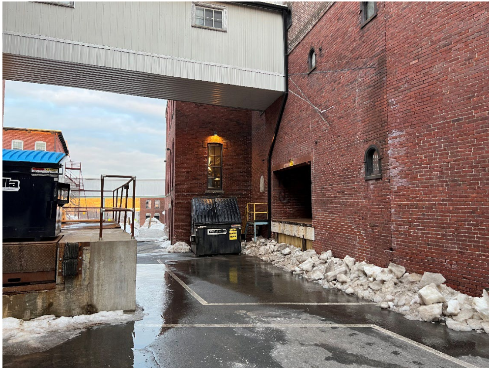
Existing Building 36 Loading Dock at End of Alleyway (Looking East)
