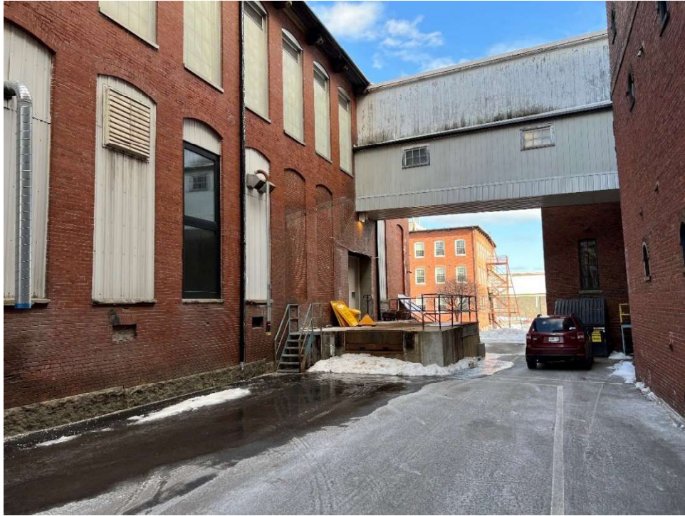
Building 13 Loading Dock in Rear Alley (Looking East)
