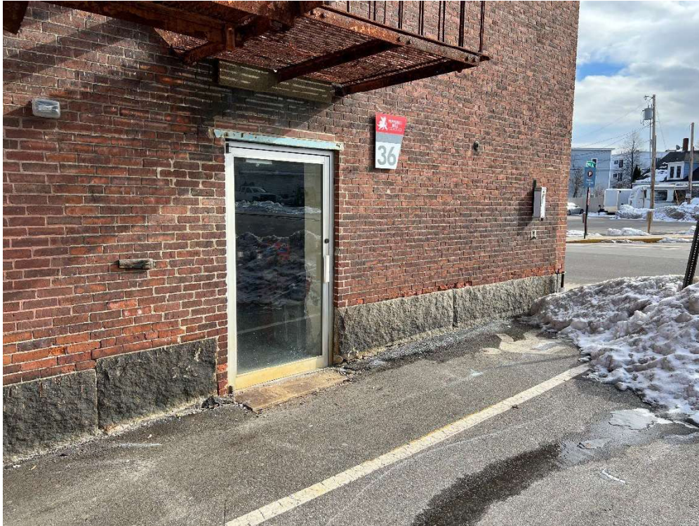
West Entrance of Building 36 (Looking Southeast)
