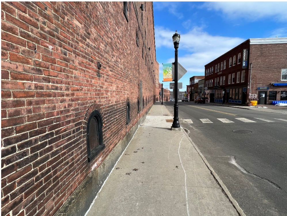
South Face of Existing Building (Looking East)
