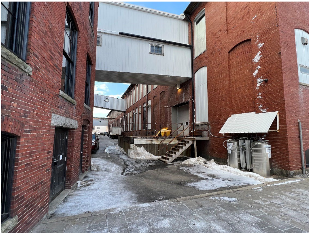
Aerial Bridge over Rear Alley (Looking West)
