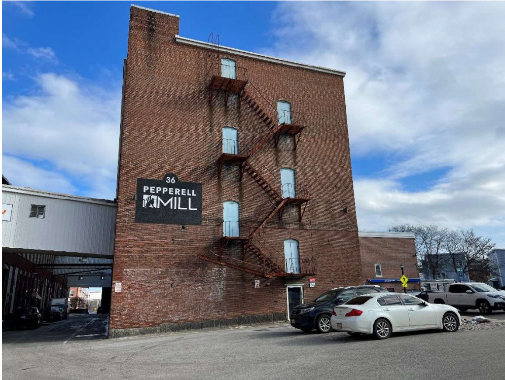
West Face of Building 36 (Looking East)
