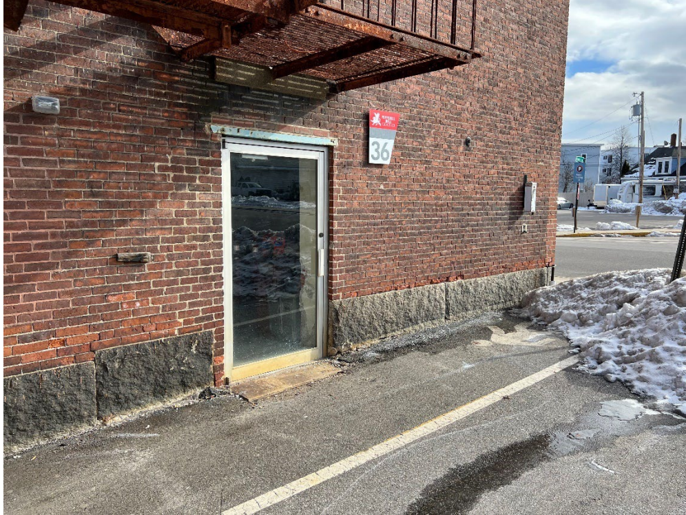
West Entrance of Building 36 (Looking Southeast)
