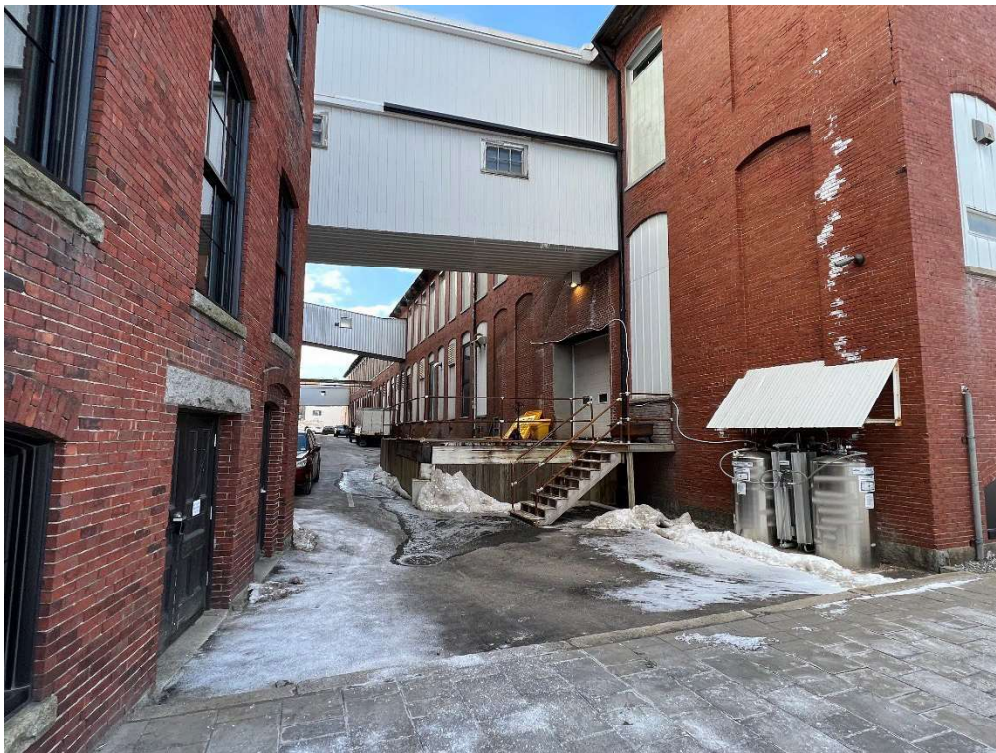
Aerial Bridge over Rear Alley (Looking West)
