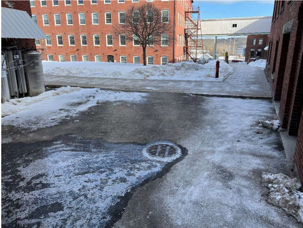
Sidewalk and Catch Basin in Alleyway (Looking East)
