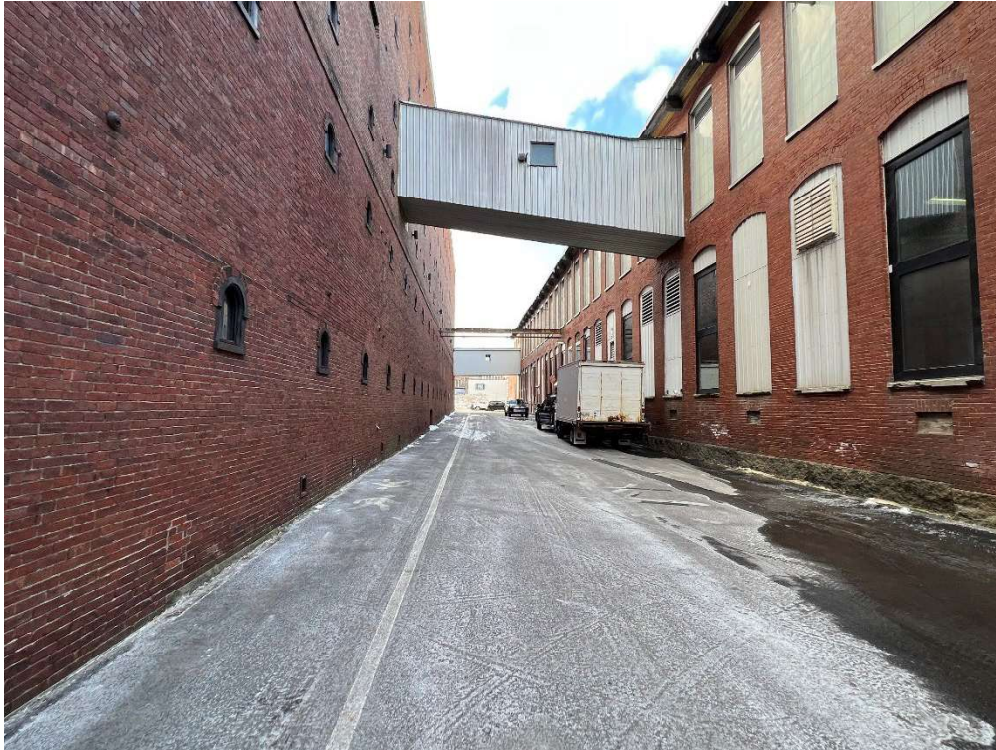
Alleyway and Aerial Bridge Adjacent to Existing Building (Looking West)
