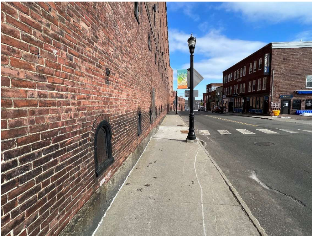
South Face of Existing Building (Looking East)
