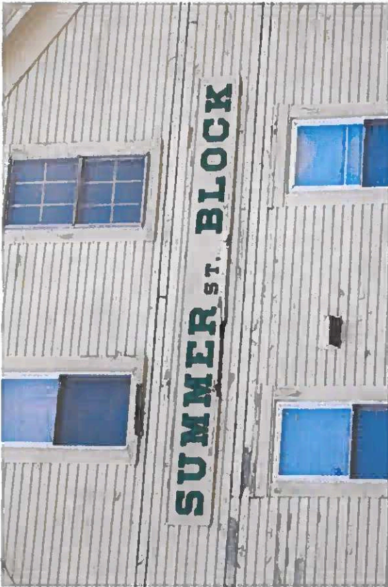
21 West Elevation - detail of historic sign
