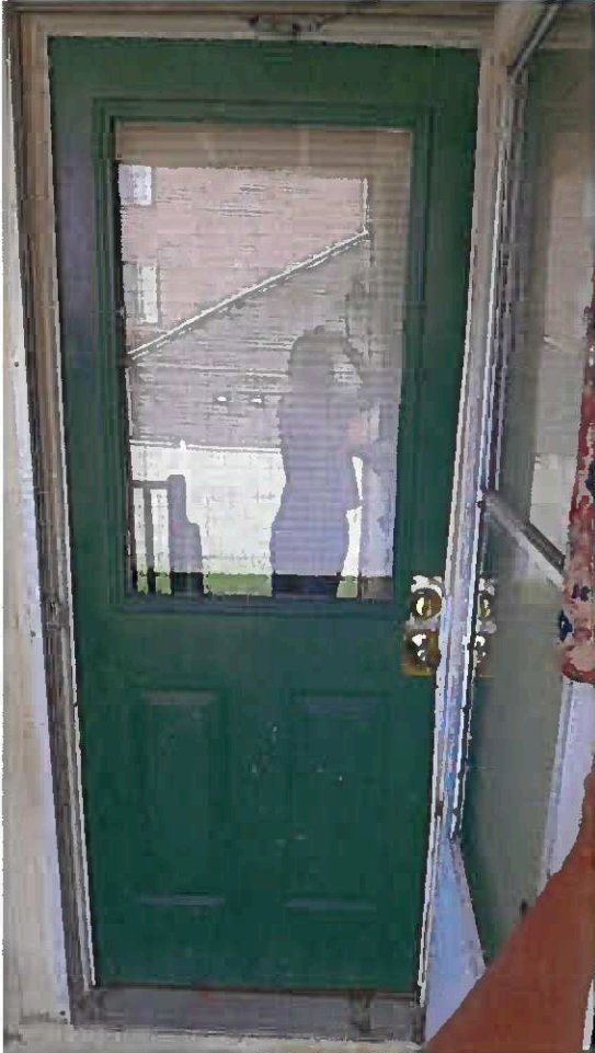
17 | Rear (North) Elevation - typical rear entrance
