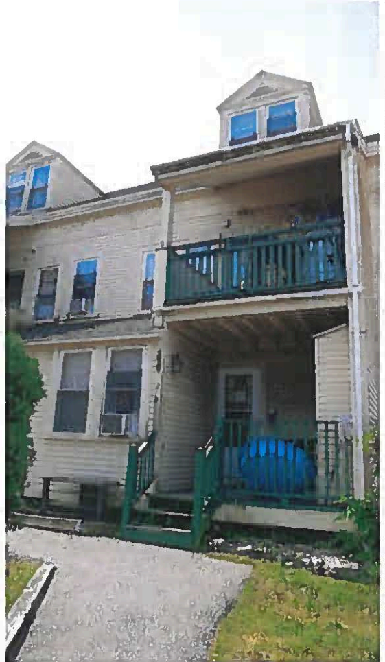
15 | Rear (North) Elevation - detail at west end
