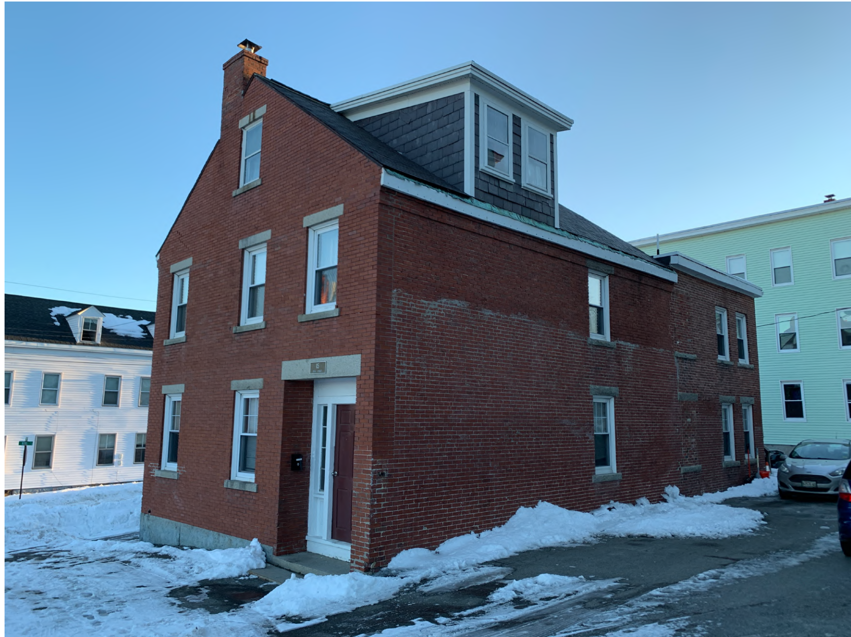
CURRENT VIEW FROM FOSS STREET
