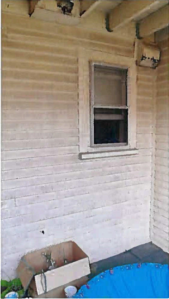
18 | Rear (North) Elevation - typical original window at rear
