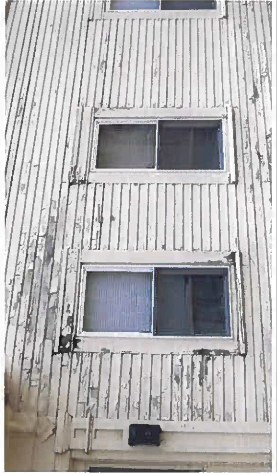
7 | Facade (south elevation) - typical first floor windows
