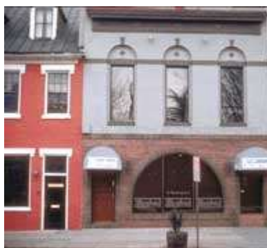
Incompatible replacement storefront and inappropriate window alteration.
