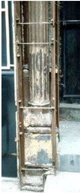
Cast iron column revealed during removal of non-significant storefront.
