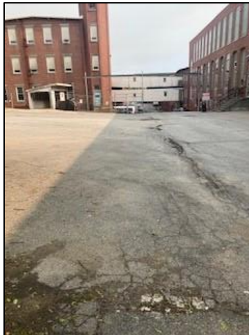
Figure 2: Laconia Street Looking North. Building 9 is at left.
