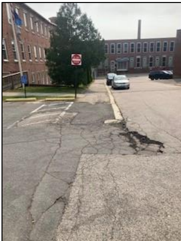
Figure 4: York Street Looking East toward Building 13
