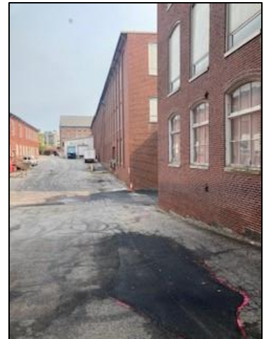
Figure 3: Laconia Street Looking North. Building 11 is at Center
