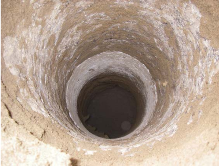
Photo 3: Bituminous & Concrete Core
