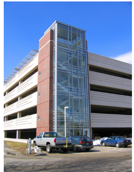
University of Southern Maine parking garage.
