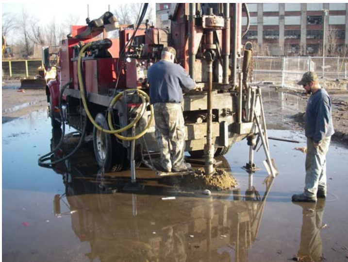
Photo 1: Truck mounted drill rig augering at B1
