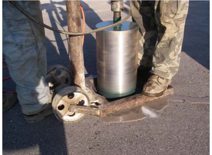
Photo 2: Concrete core drilling at B2
