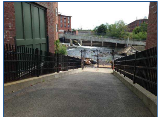
Photo 5: View of Ramp to Fall Plaza Area.
