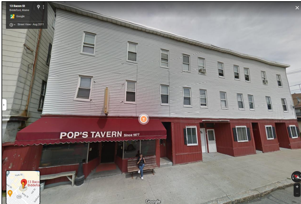
Source: "13 Bacon Street, Biddeford, Maine." 43.49° N, 70.45° W. South Elevation. Google Earth Street View . Imagery Date: 08/2011. Accessed Date: 06/30/2022.
