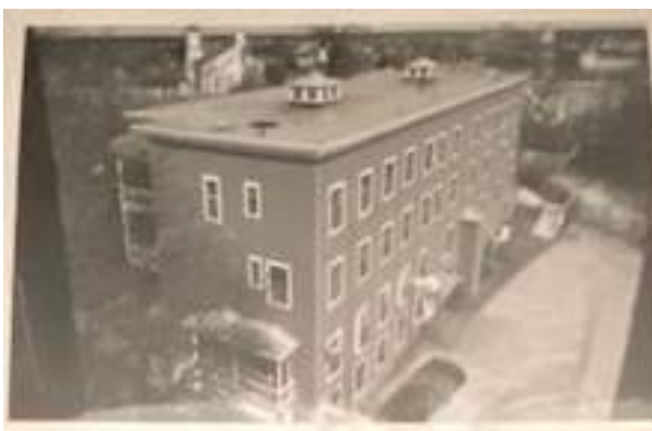
Original Convent on proposed site prior to fire
