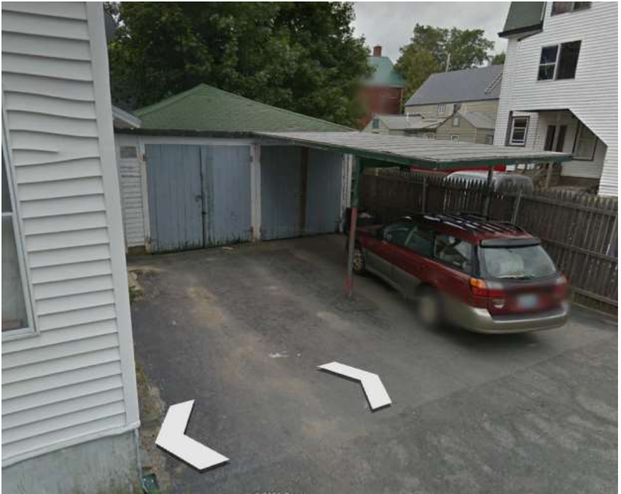
Source: "20 Wentworth Street, Biddeford, Maine." 43°29'30.66" N 70°27'42.85" W. Google Earth Street View. Imagery Date: 8/2011. Accessed Date: 7/9/2020. Rear garage as seen from Wentworth Lane
