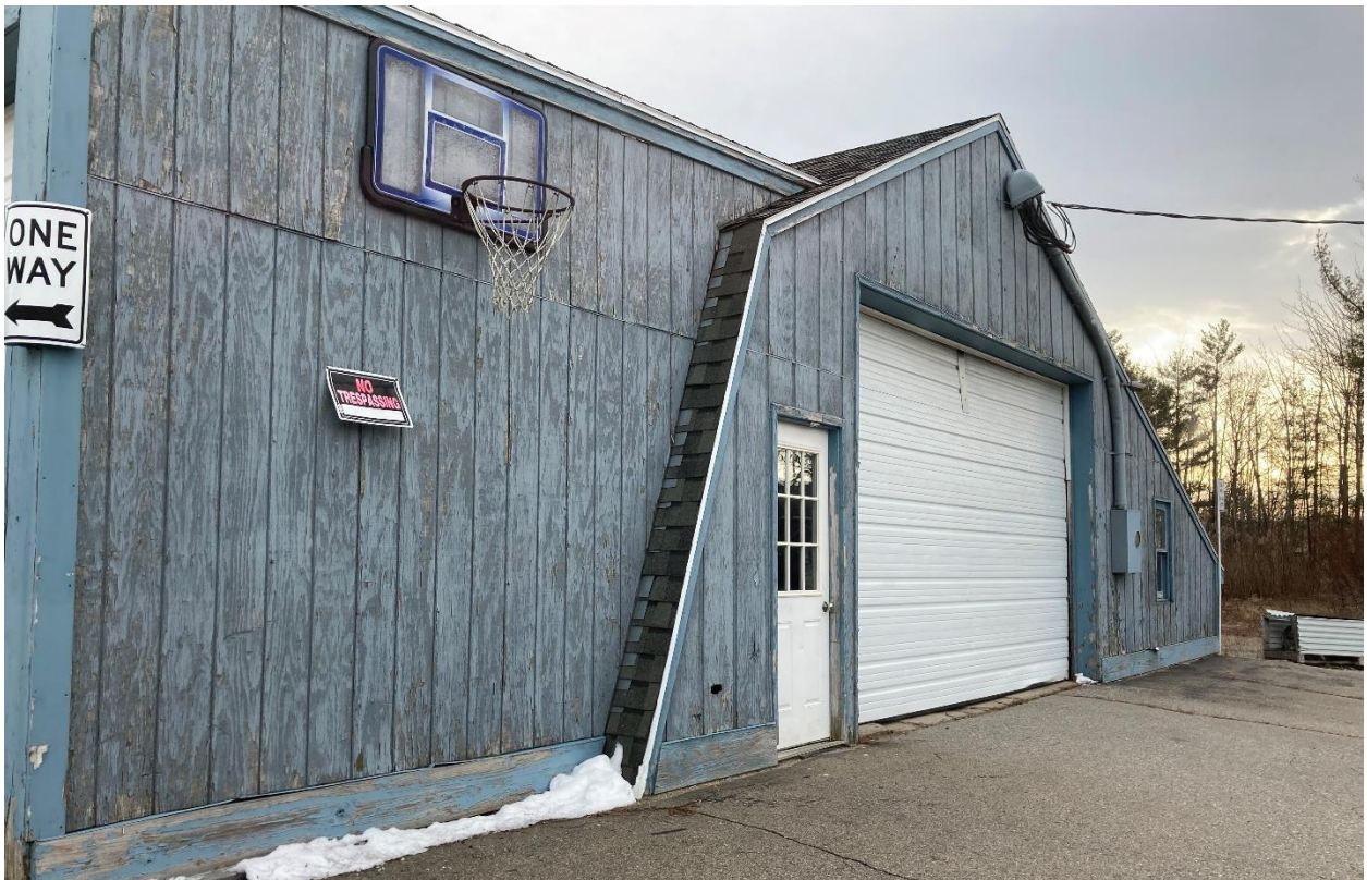
Front entrance to storage garage
