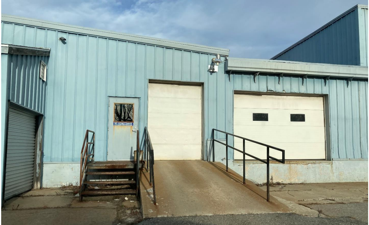
Loading dock and dolly ramp
