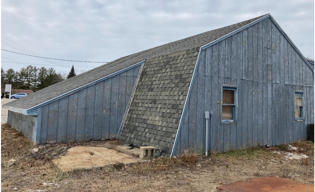
Rear of storage garage
