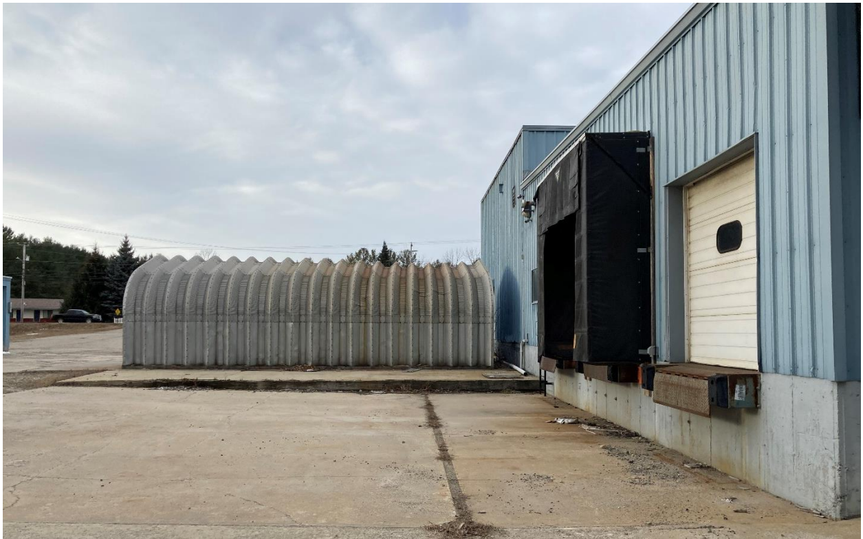
Loading docks and Quonset hut
