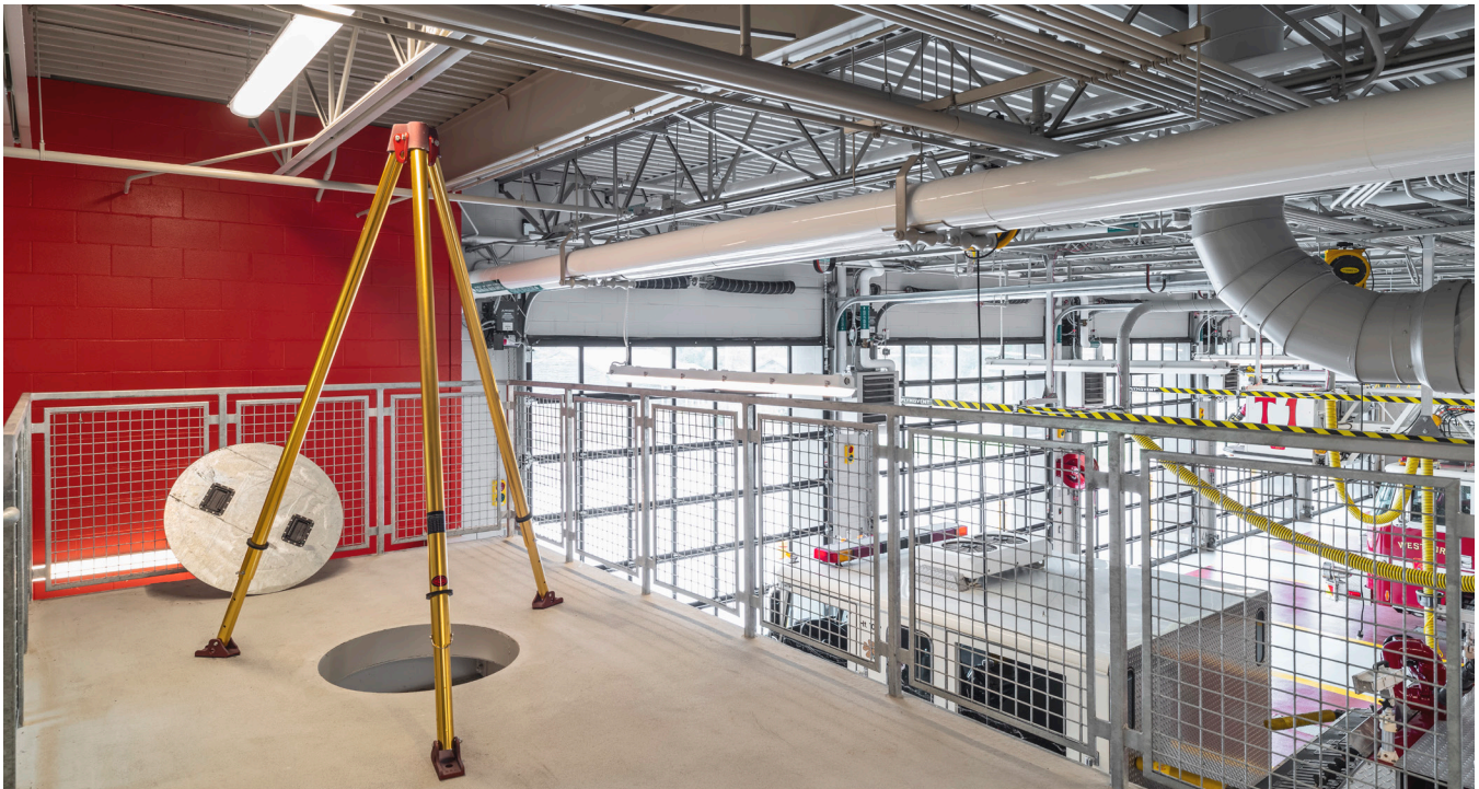
Fire Headquarters | Westford, MA
