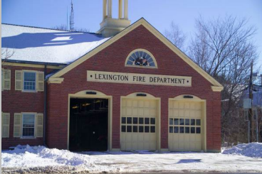
Lexington Fire Station
