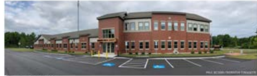
Yarmouth Public Safety Building
