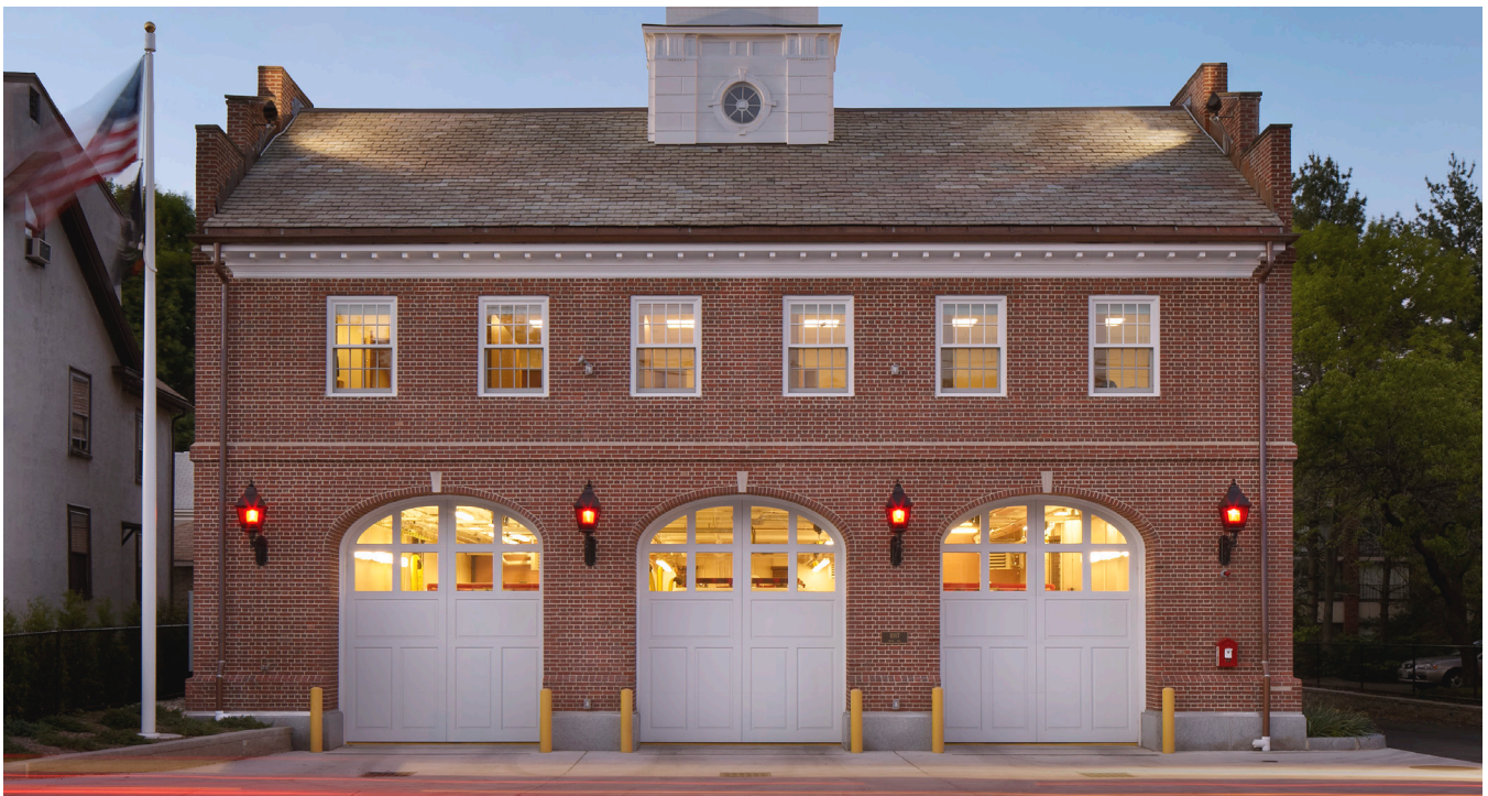
Highland Fire Station | Arlington, MA
