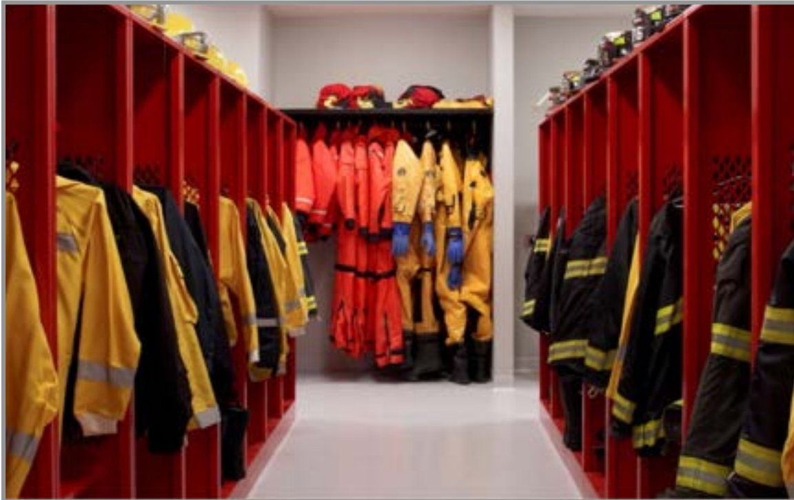
Turn Out Gear Room: Saco's design has access to bays, walk-in decontamination shower and Slide Pole.
