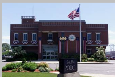
Salem Police Station
