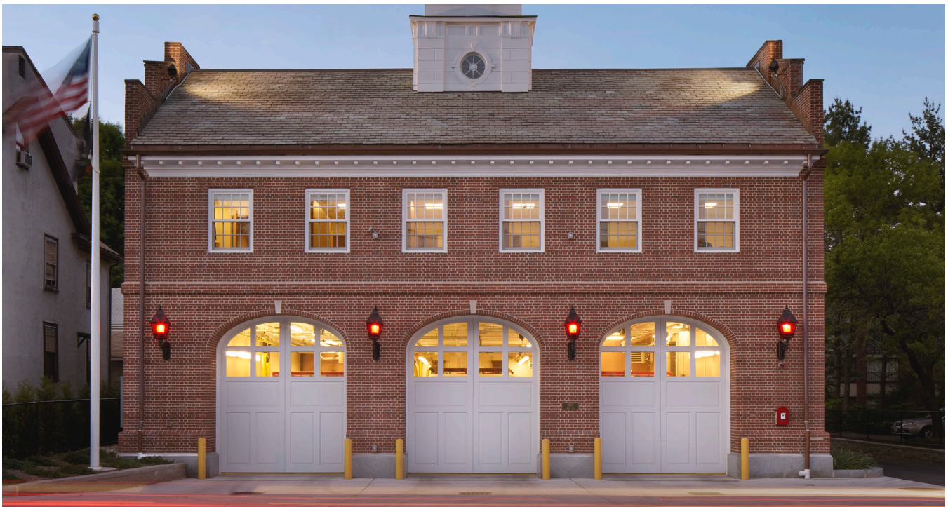
Highland Fire Station | Arlington, MA
