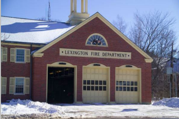
Lexington Fire Station
