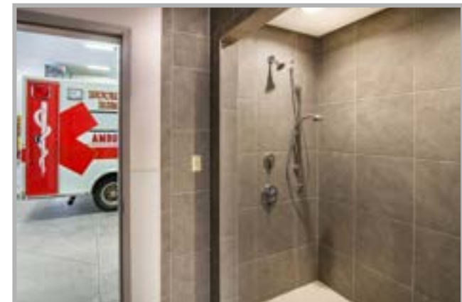
Decontamination Room: A walk-in decontamination shower allows for stretcher boards and other large items to be washed.
