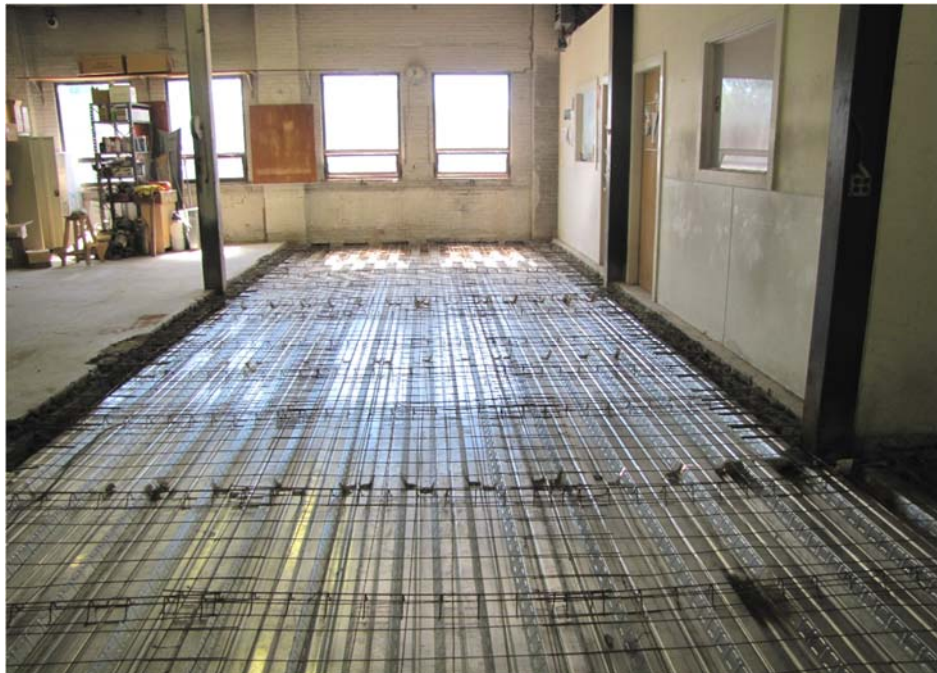
DPW Garage Structural Modifications
