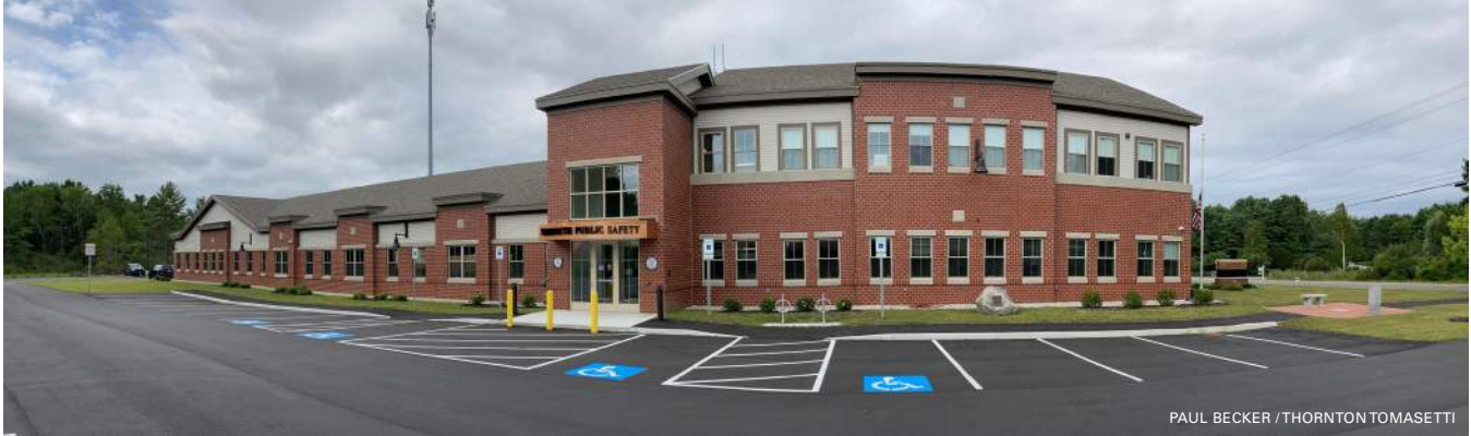
Yarmouth Public Safety Building
