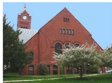
Winchester Town Hall (Historic)
