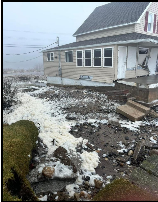
Photo 3: 67 Fortunes Rocks Road facing northwest
