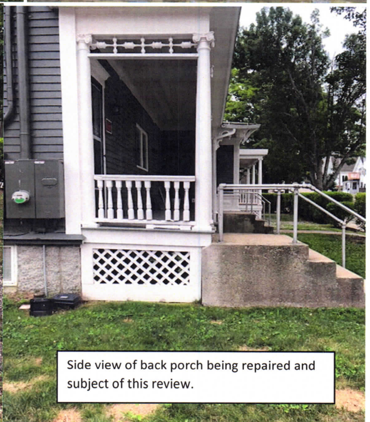
Front porch completed previously per NPS guidelines and approval. Skirting on back porch to match this.
