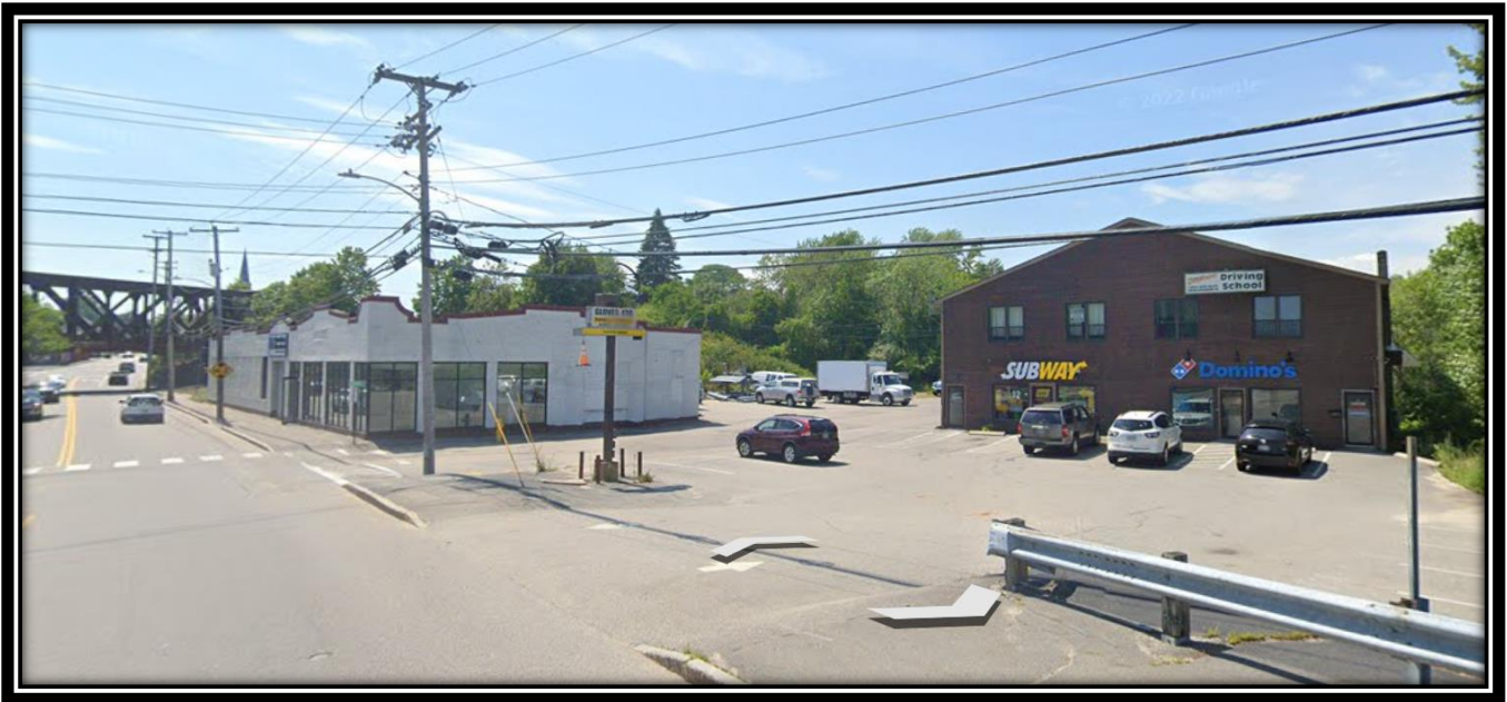
View of the two (2) buildings at Diamond Street and Elm Street proposed for demo / redevelopment
