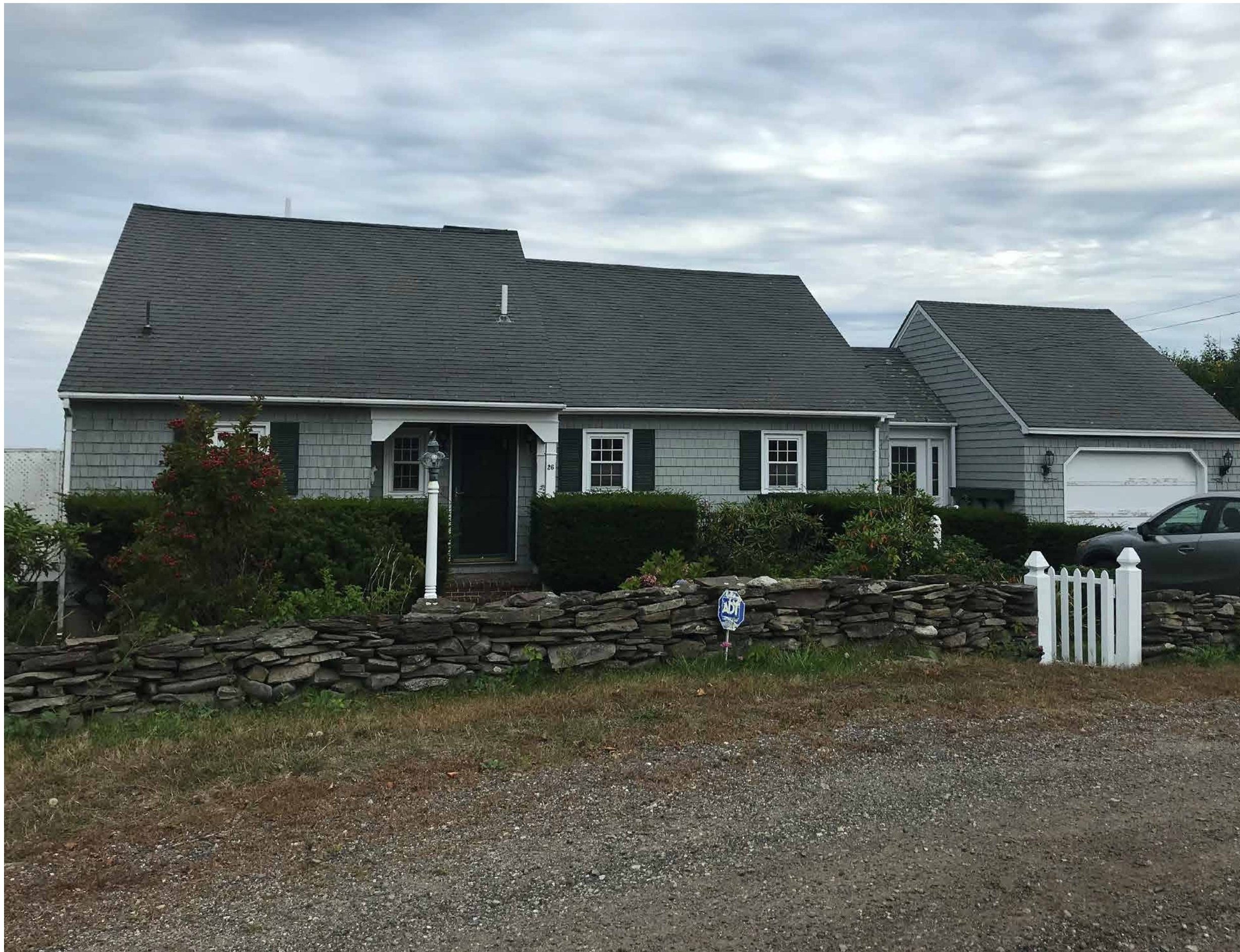
EXISTING BUILDING - STREET SIDE
