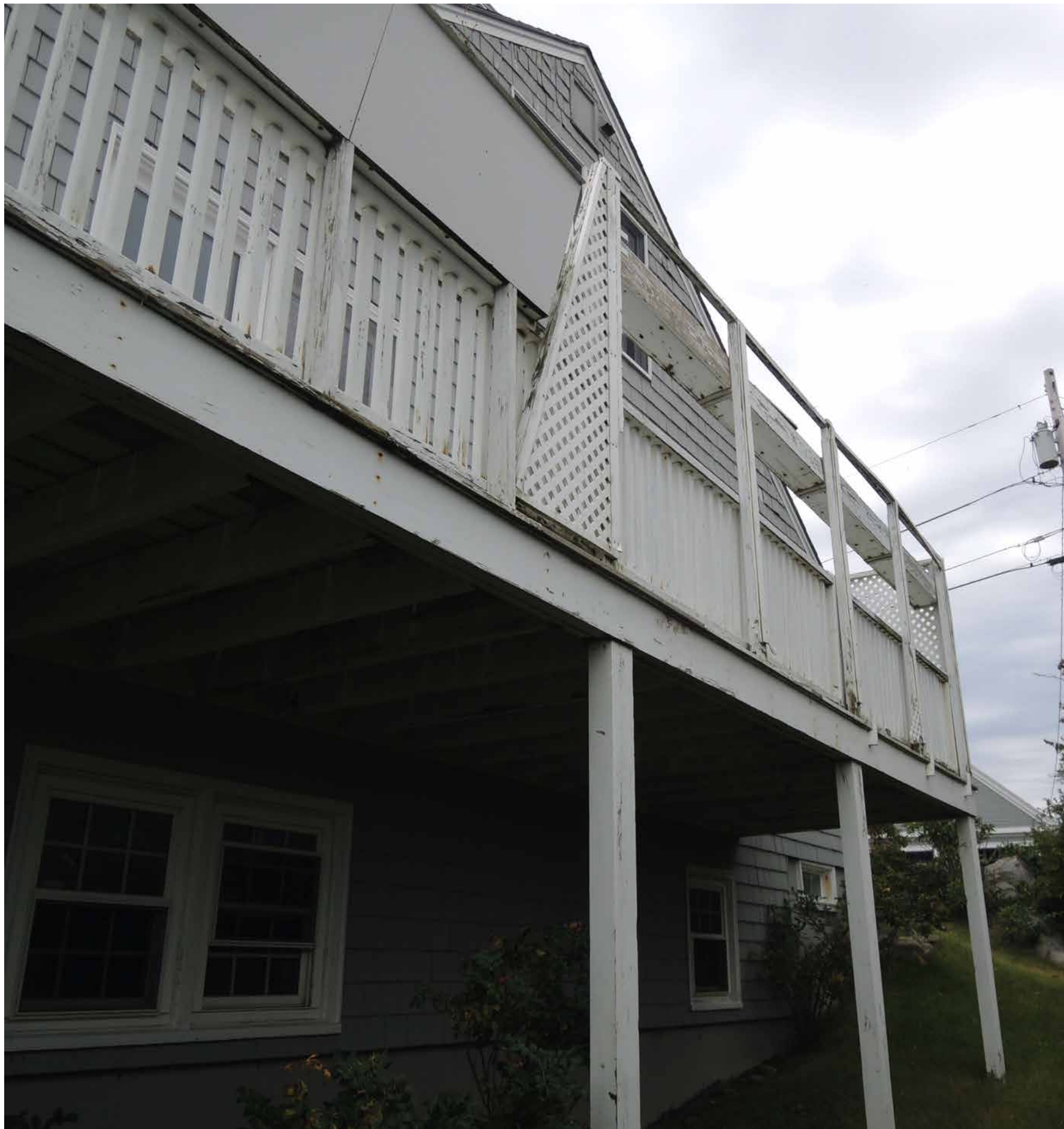
EXISTING NORTH SIDE YARD/DECK
