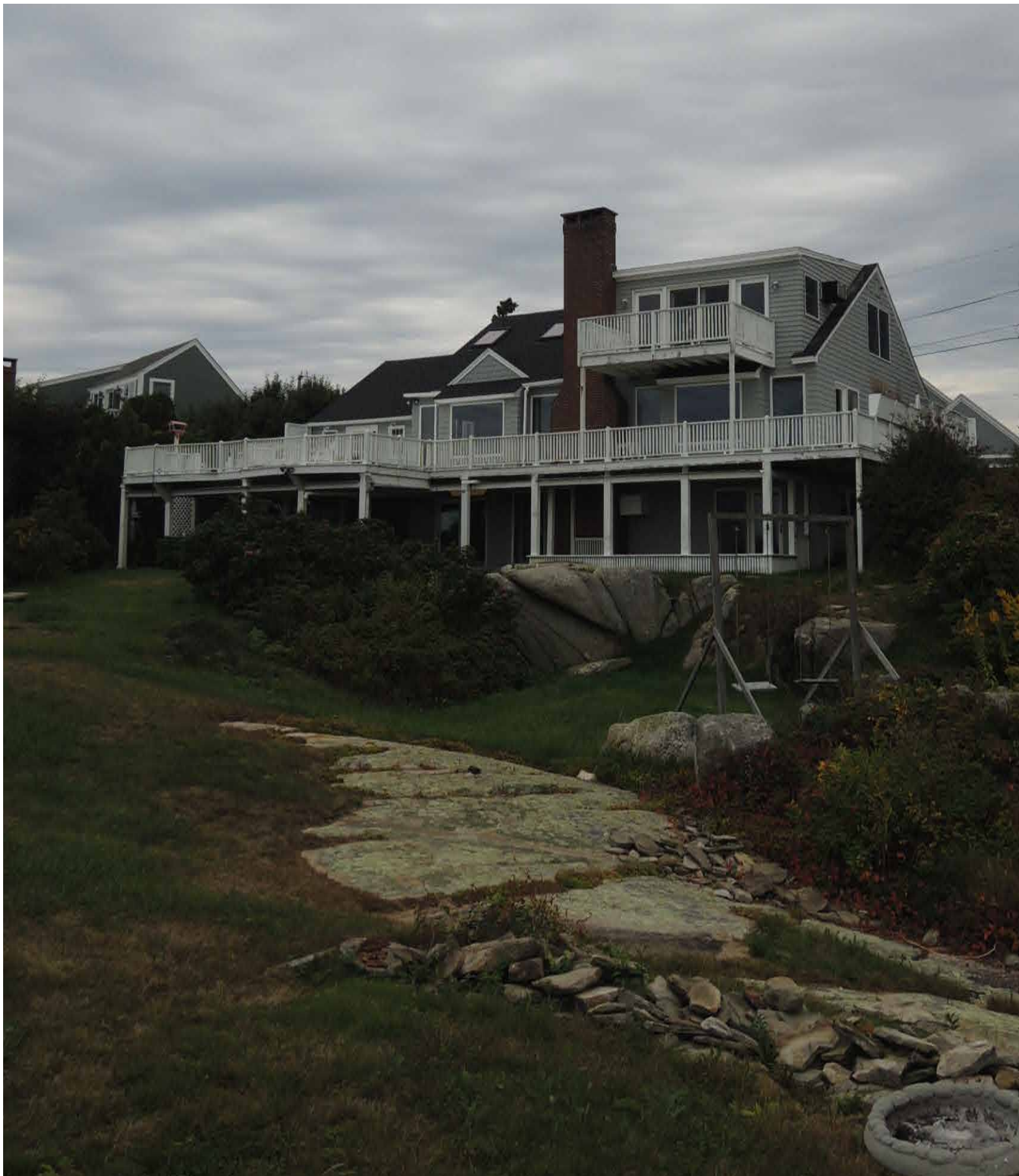
EXISTING BUILDING - FROM OCEAN
