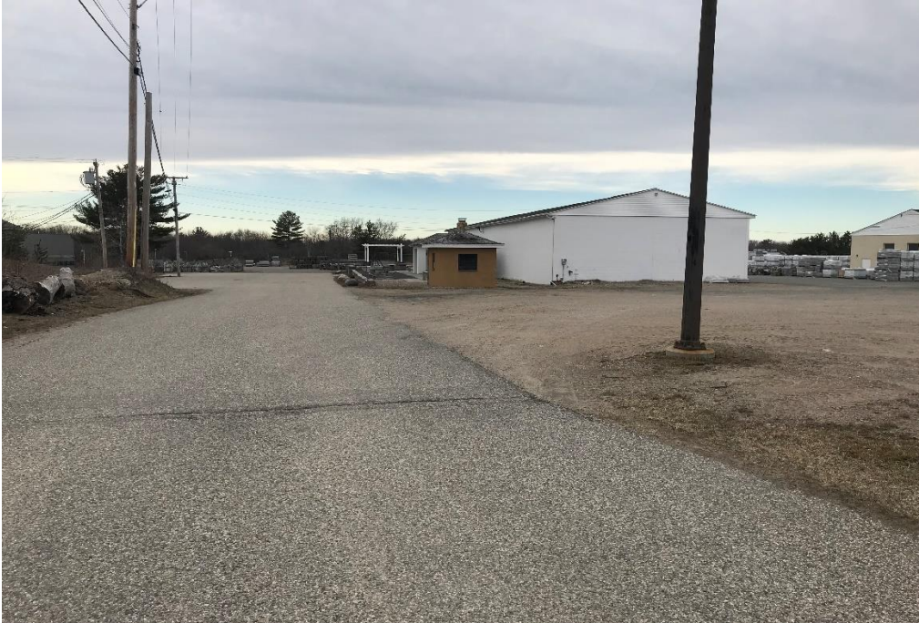
Photo 4: Looking northwesterly towards existing building, demonstration area, and parking.
