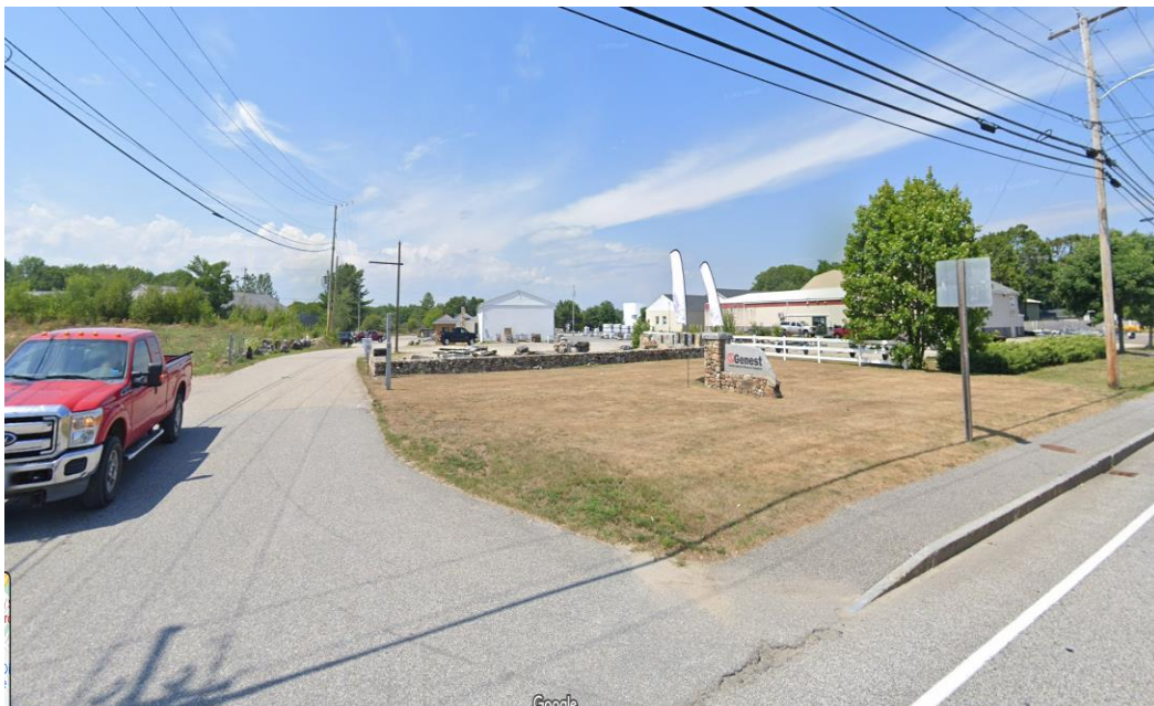
Photo 2: Travelling north on Elm Street (US Route 1), site entrance on the left. Existing face of white building where building addition is proposed.
