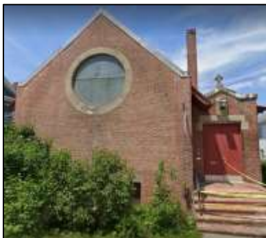
Existing Front Entry
