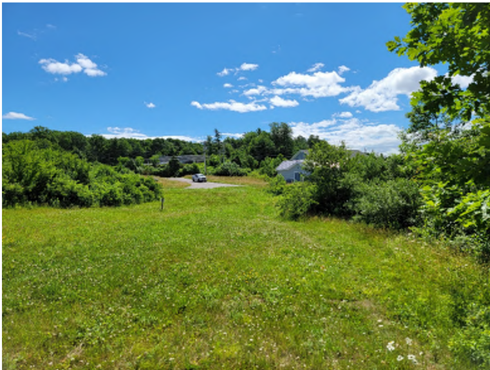
Drive and Pump Station from Sewer Easement (Looking East)
