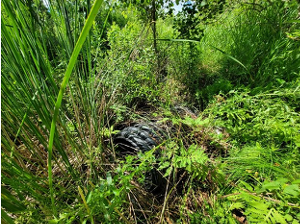
Outlet of Pond (Looking South)
