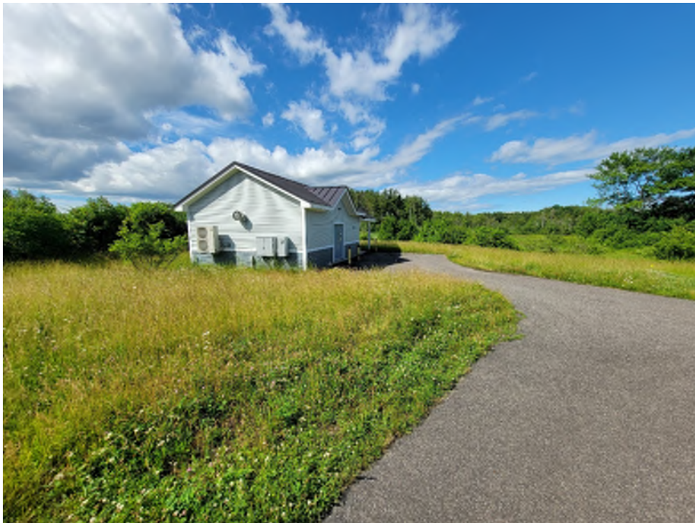
Maine Water Pump Station Building (Looking Southwest)
