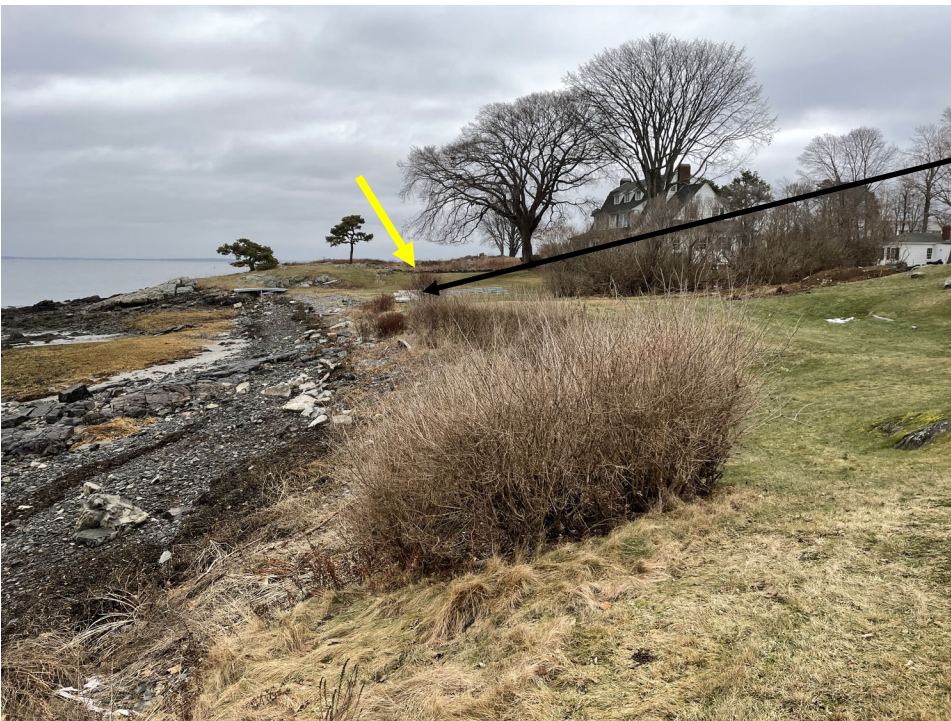
Shoreline stabilization ends at large shrub, existing grade rises above elevation 10.5—11
