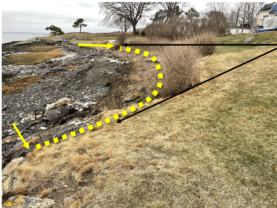
Area of shoreline erosion, from pier to shrub in the far distance. Approximately 130 linear feet of shoreline stabilization.
