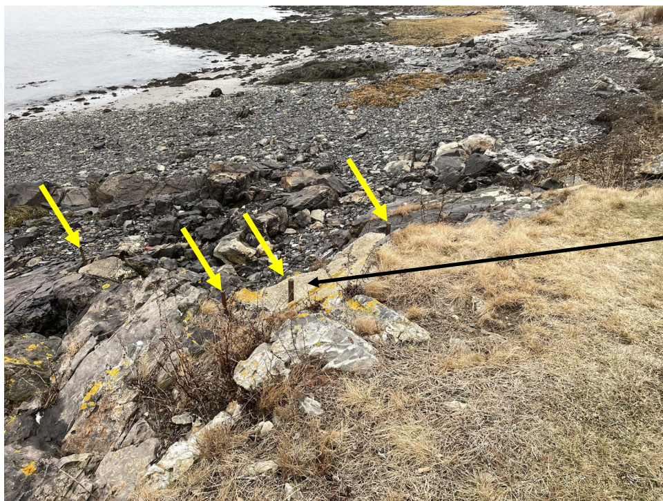
Pins to mount existing seasonal pier, ramp and float.
