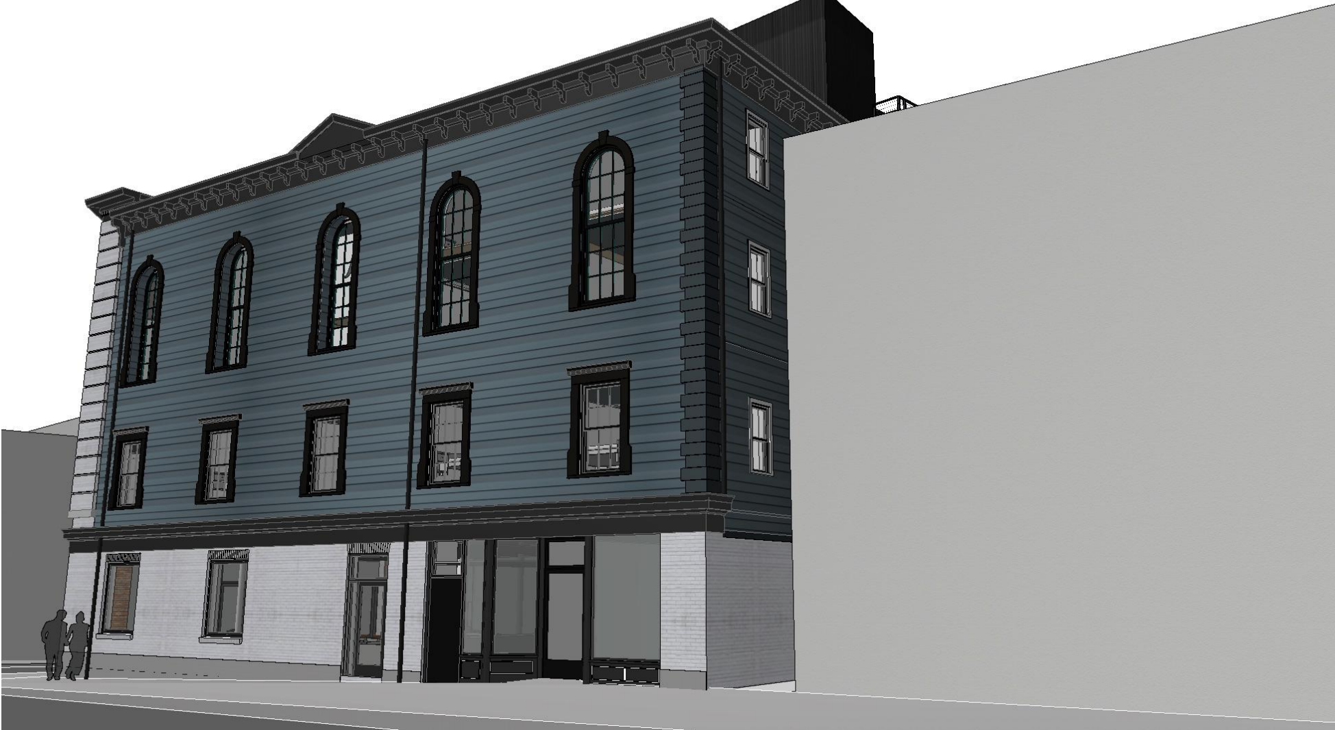
4 - ACROSS BACON STREET
