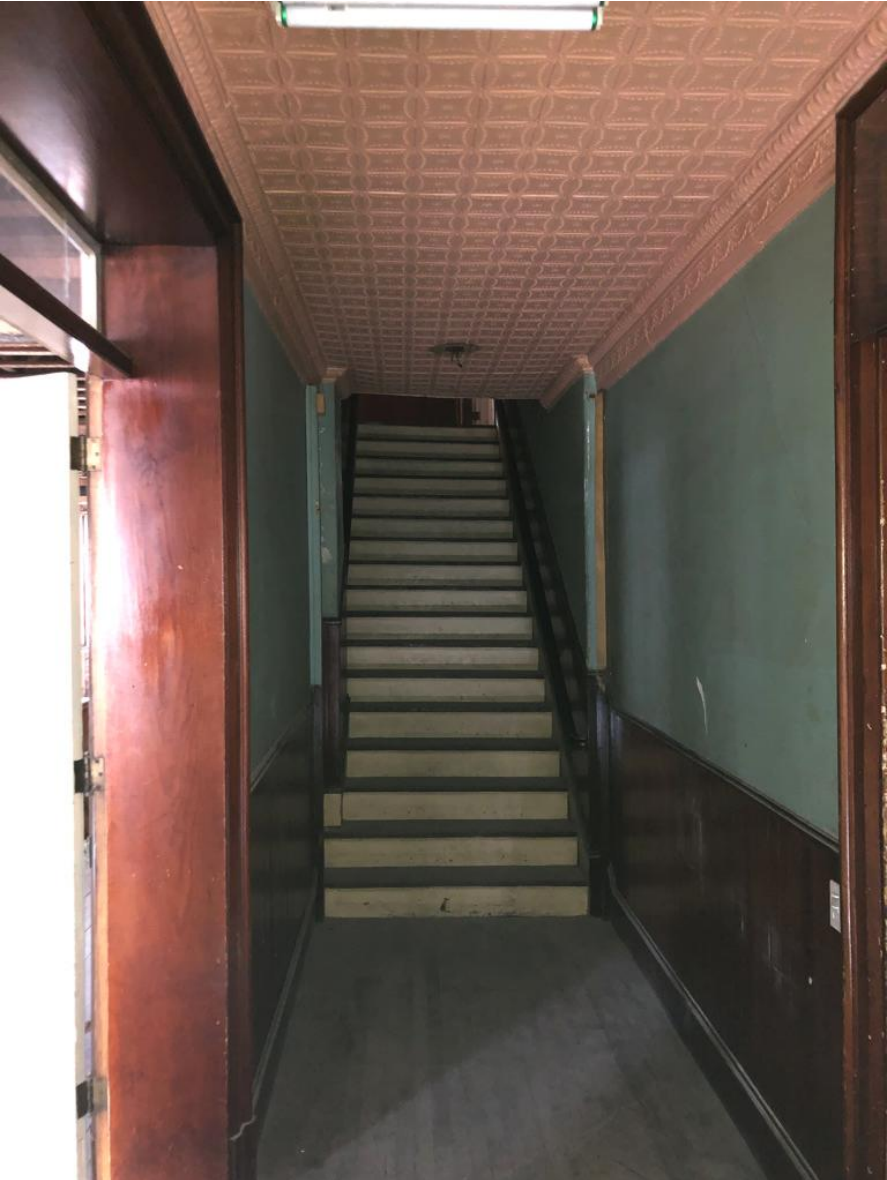
2ND FLOOR - EXISTING STAIR UP TO 3RD FLOOR
