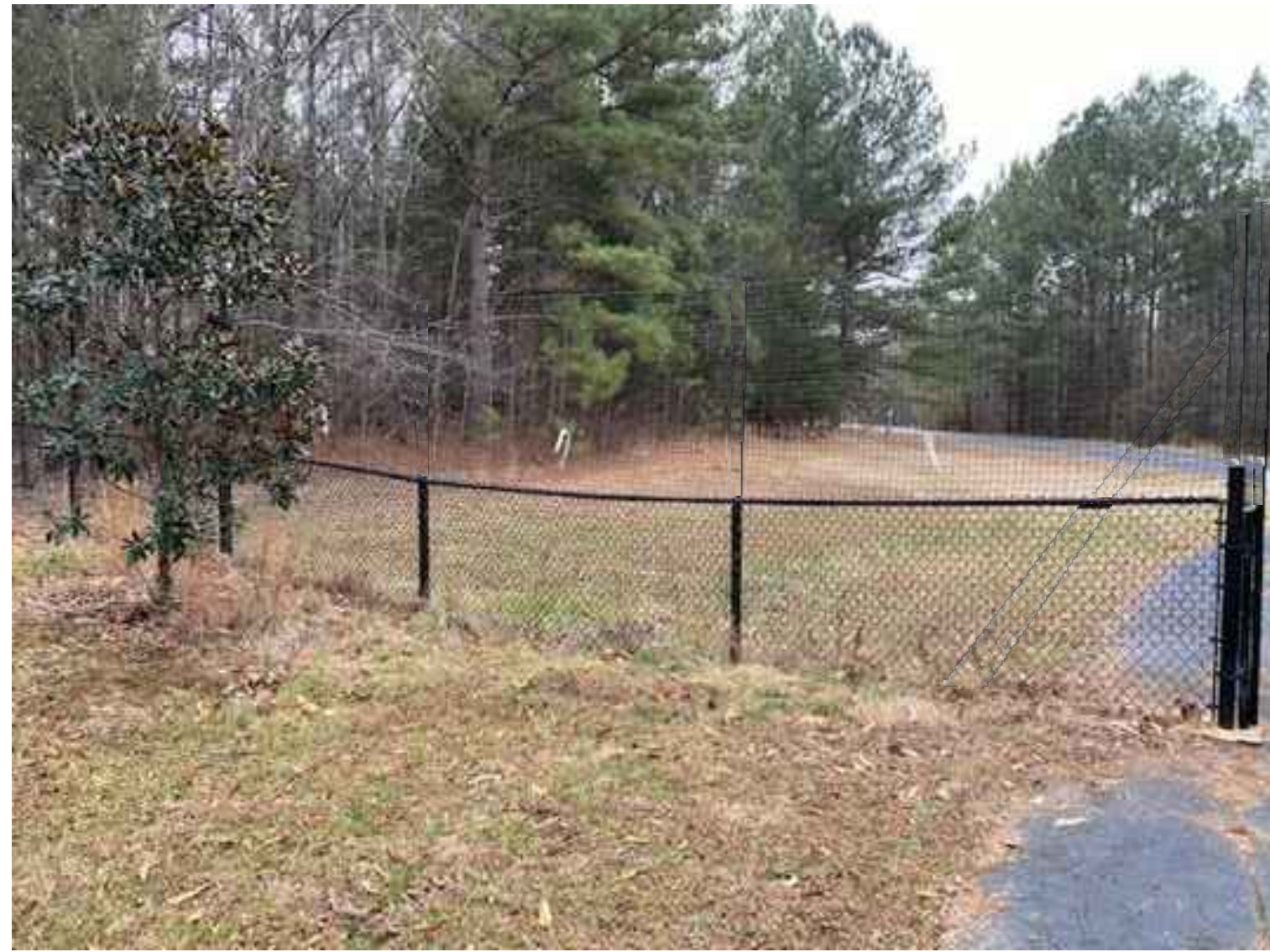
SIMILAR INSTALLATION CRITTER FENCE
