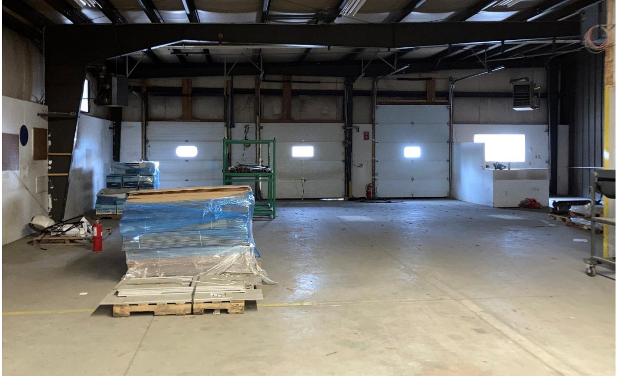
Loading dock area
