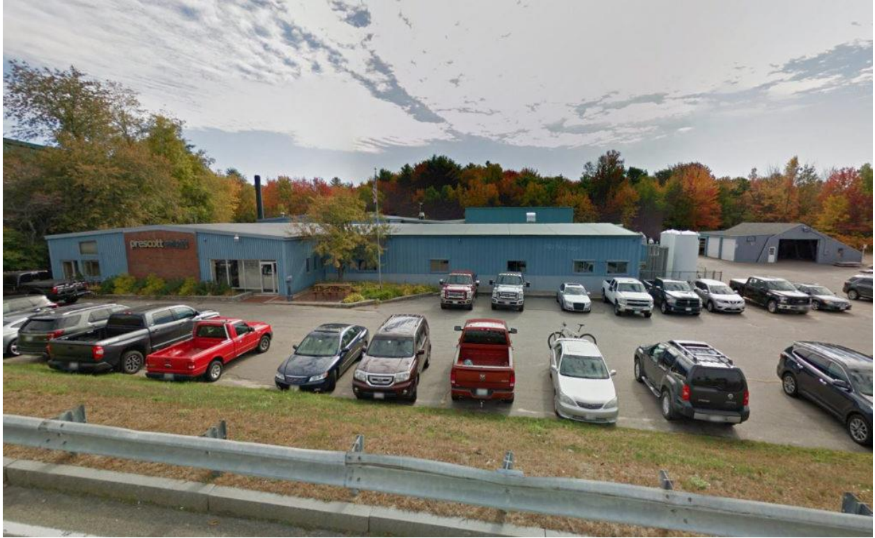
View of building from Elm Street
