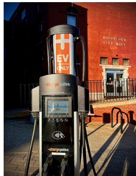
EV Charing Station. PhotoVoice Contest 2023 Entry.
