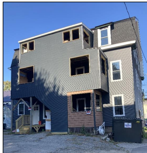
Rear of building today. Note new rear door lower left of image
