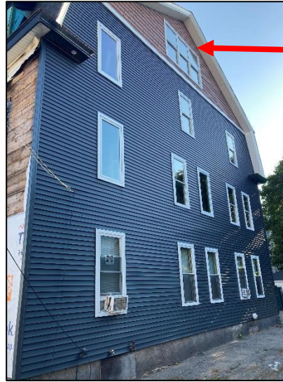
South side of building
