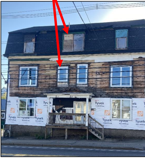
Front of building (west side)
