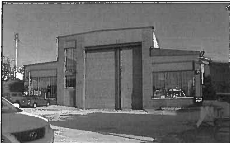
Portland Company Erecting Building Portland, Maine completed 1914
