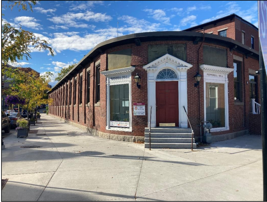
Rear of the project property looking east from Lincoln Street:
