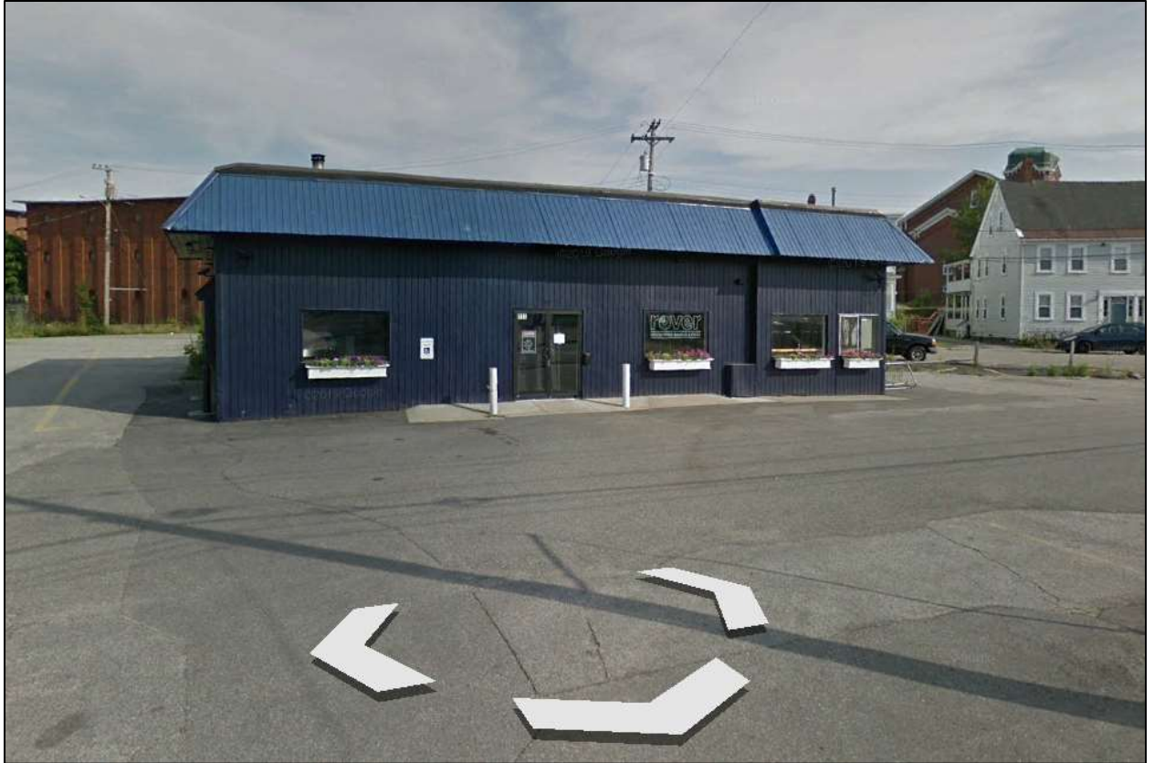
Source: "111 Elm Street, Biddeford, Maine." 43°29'43.78"N 70°27'27.32"W. Google Earth Street View. Imagery Date: 07/2018. Accessed Date: 10/05/2020.
