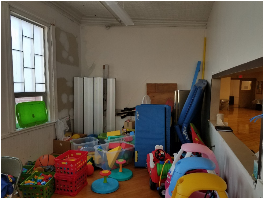
Picture #4 – Proposed Boiler Room Interior
