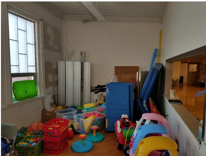
Picture #4 – Proposed Boiler Room Interior
