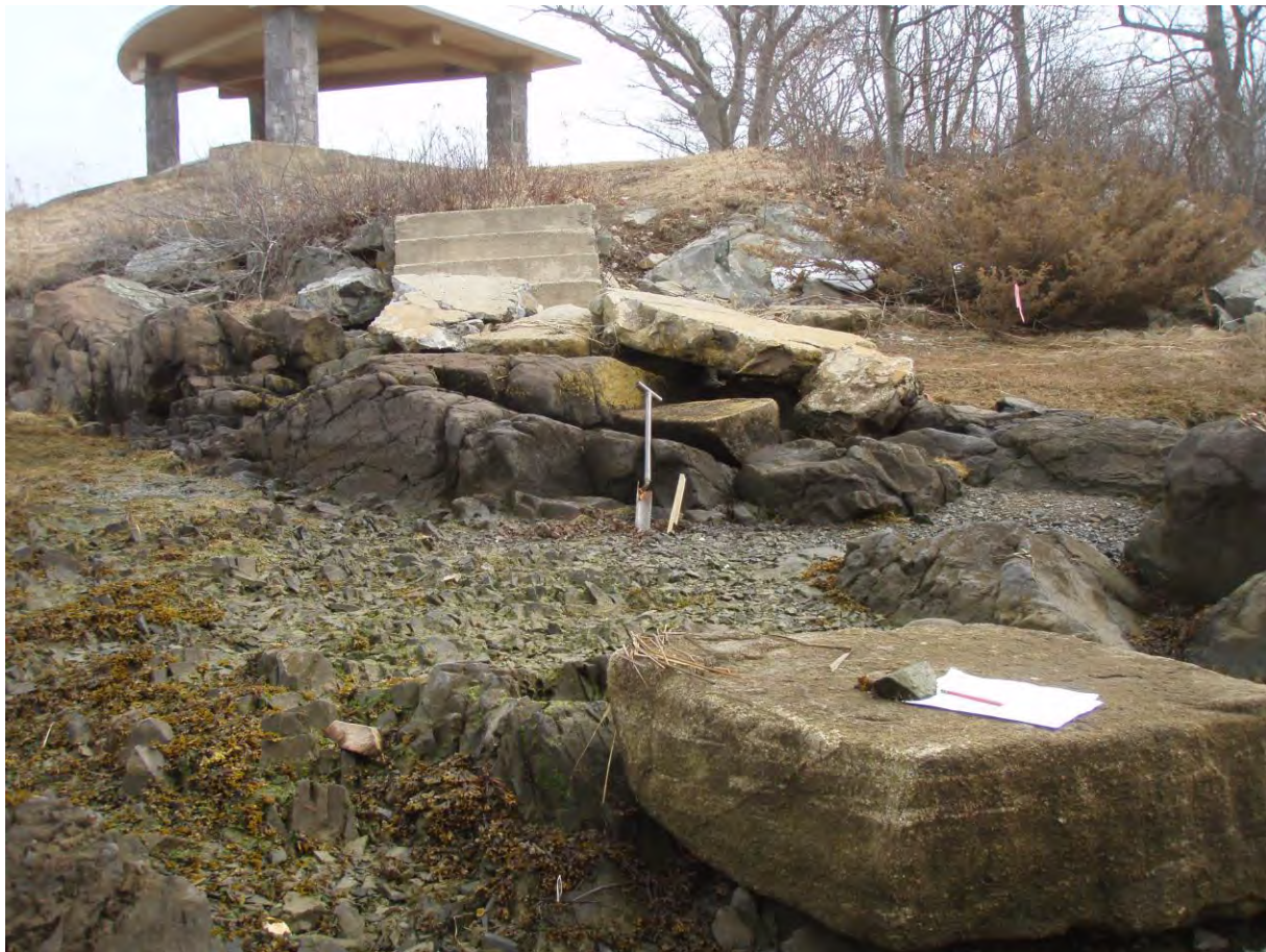
Photograph One. Note the remnant stairs and concrete materials from past pier locations and the small, isolated wetland vegetation ( Spartina alterniflora ) colony located in the upper right below the pink wetland flag. Photograph date: 03/13/2023.
