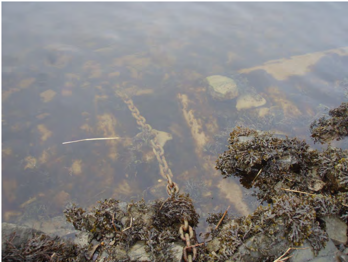
Photograph Seven. Photograph of an old chain and existing cribwork from a past pier just westerly of the proposed pier location. Photograph date: 03/13/2023.
