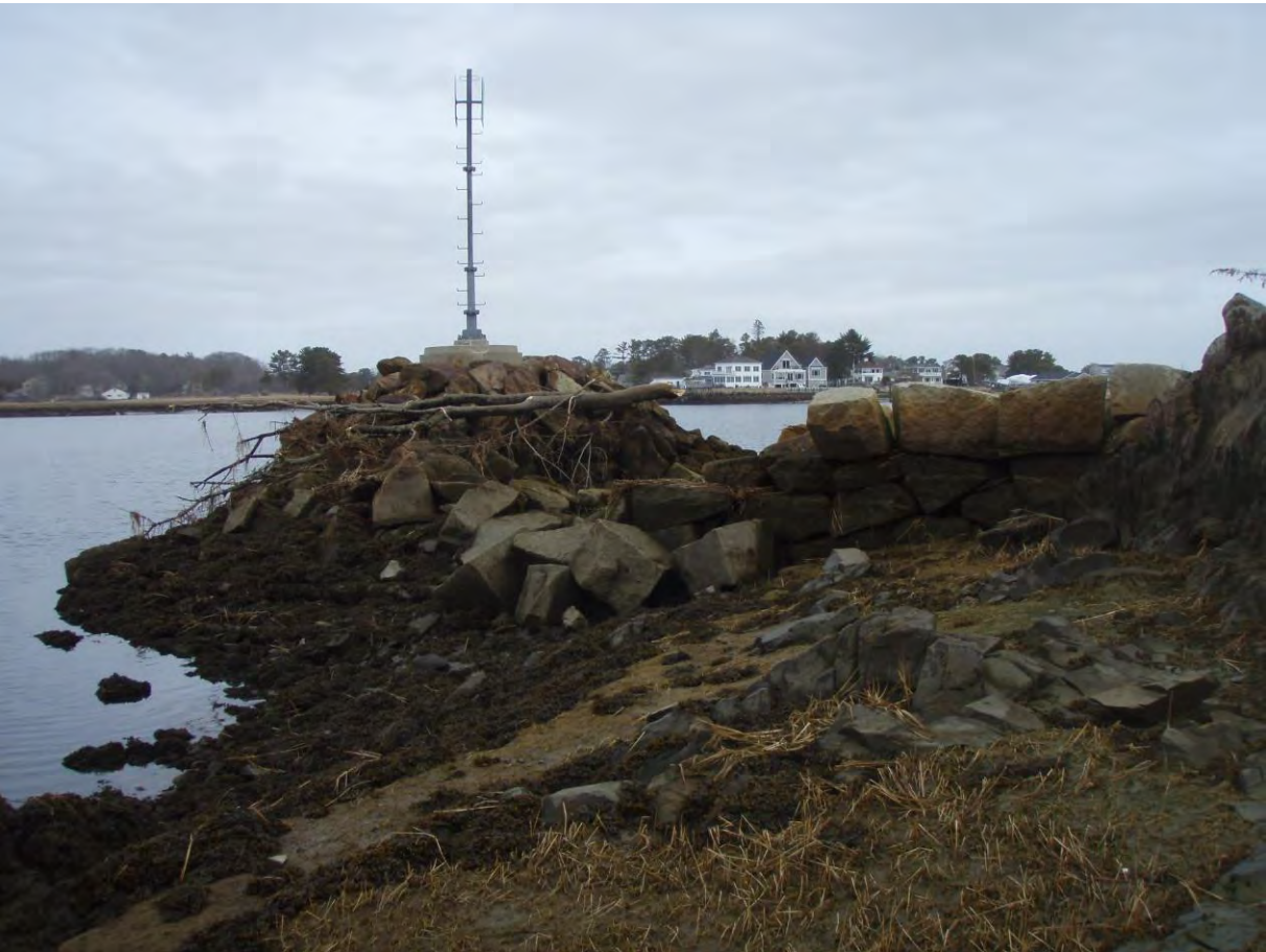
Photograph Ten. Easterly view from the proposed pier location toward the existing seawall and navigation marker with Camp Ellis in the background. Photograph date: 03/13/2023.
