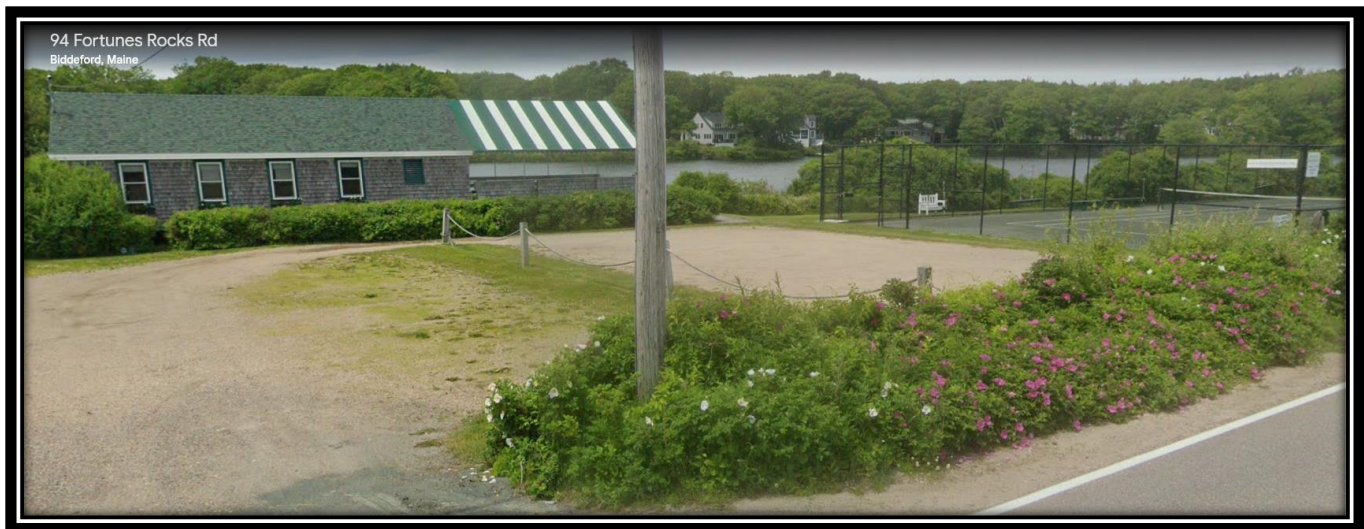
94 Fortunes Rock Road – Existing Conditions
