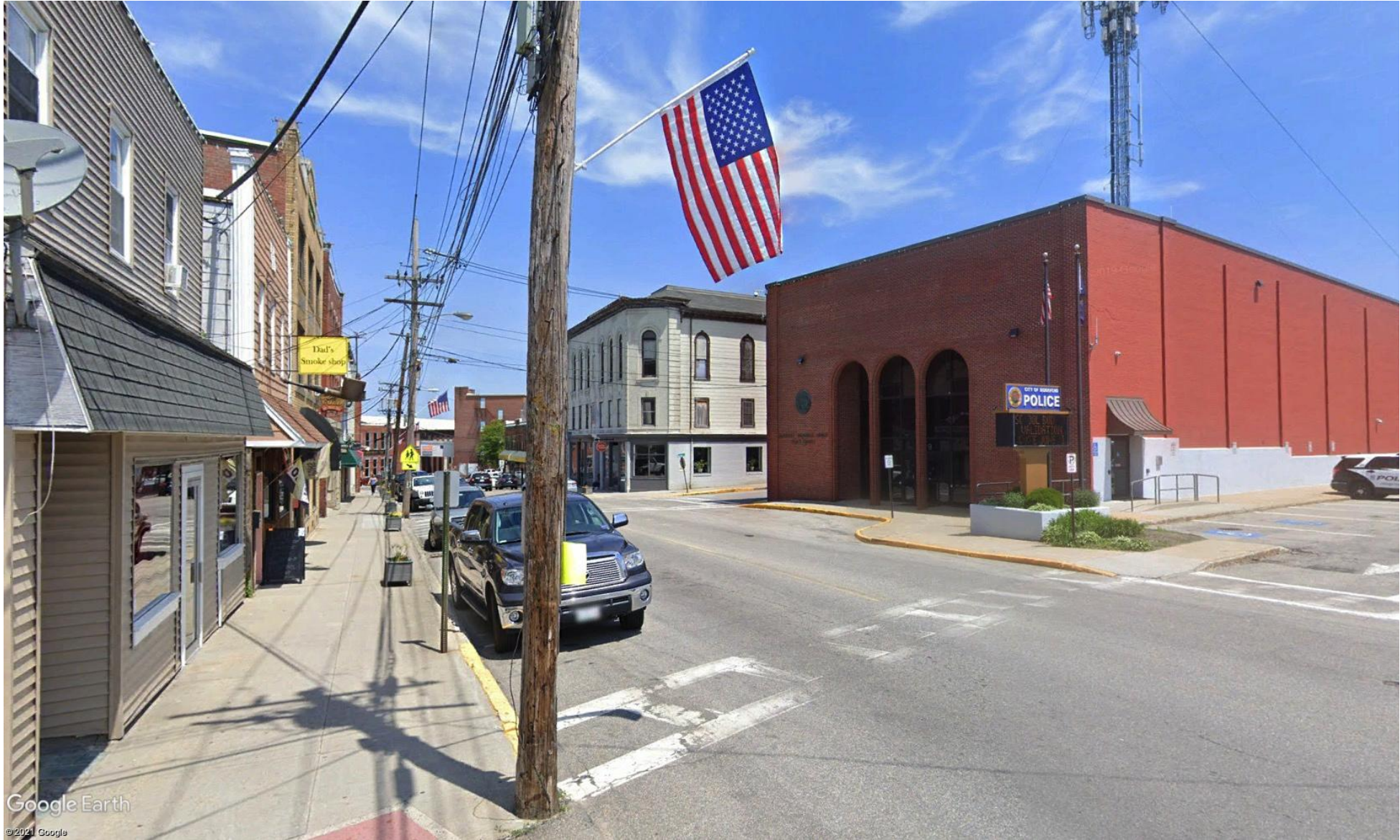
GOOGLE STREET VIEW - CORNER OF ALFRED AND FRANKLIN
