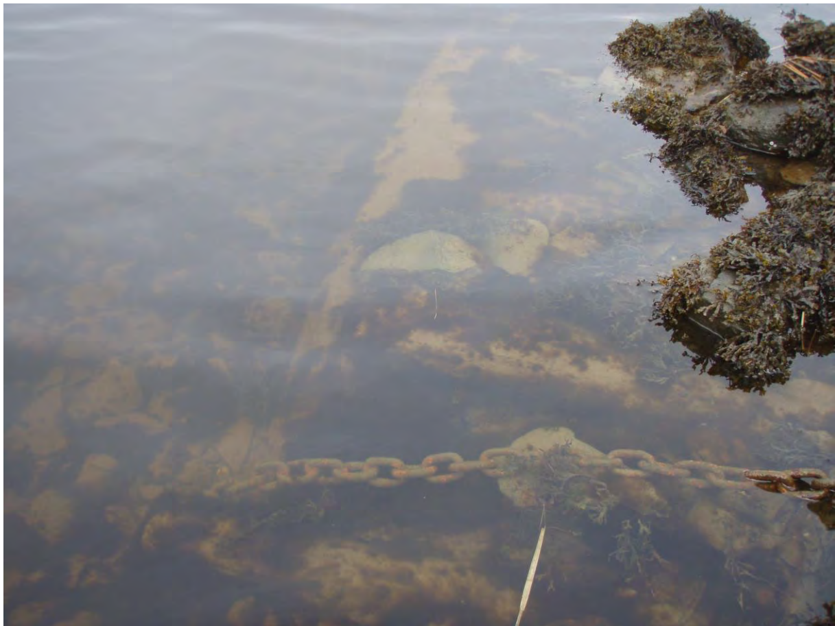
Photograph Eight. A closeup view of the existing cribwork that is exposed to this below the low tide line. Photograph date: 03/13/2023.
