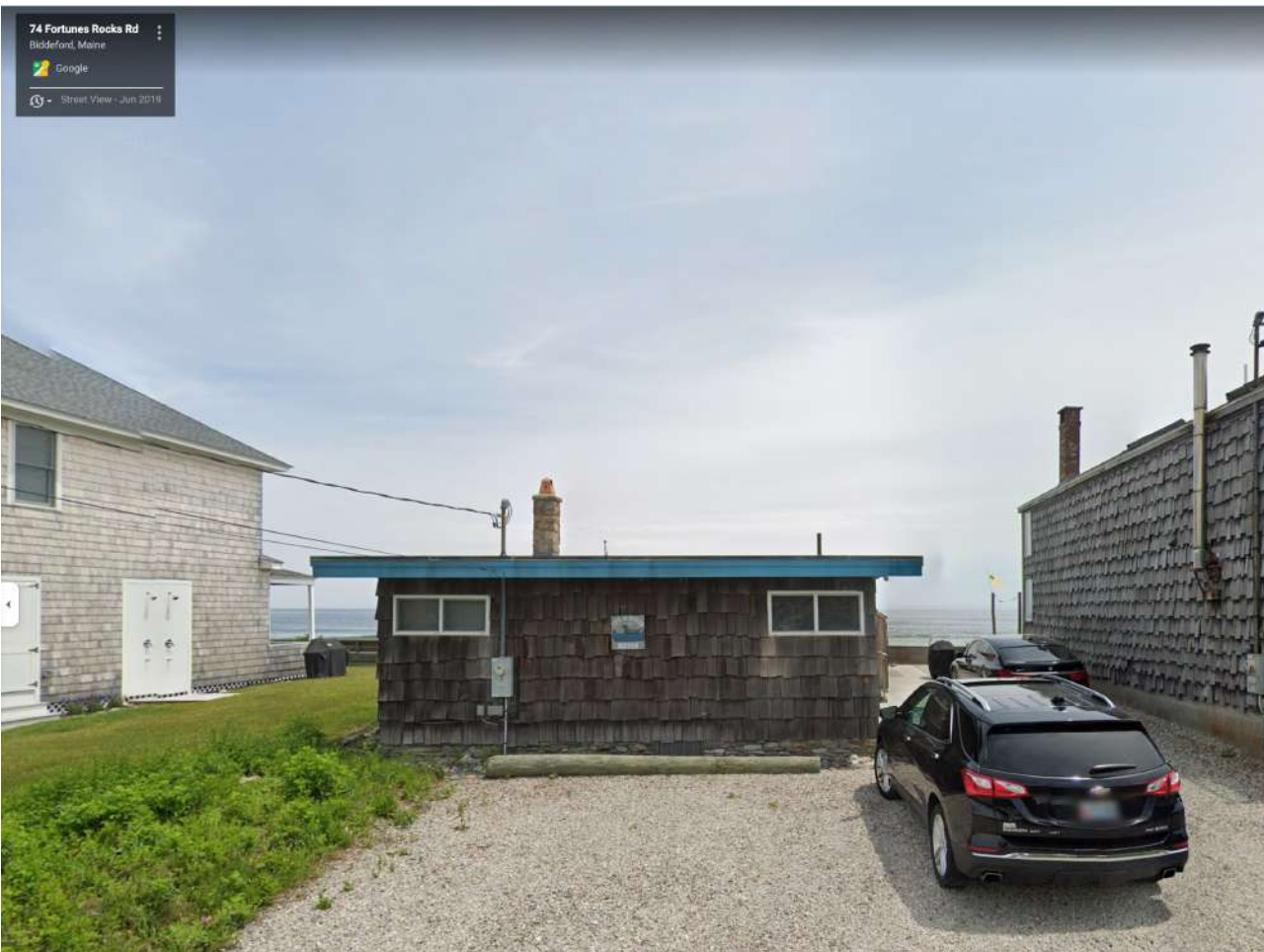
EXISTING HOUSE FROM ROAD
