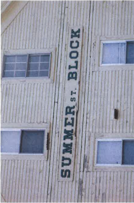
21 | West Elevation - detail of historic sign
