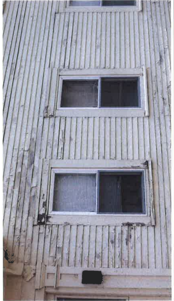
7 | Facade (south elevation) - typical first floor windows
