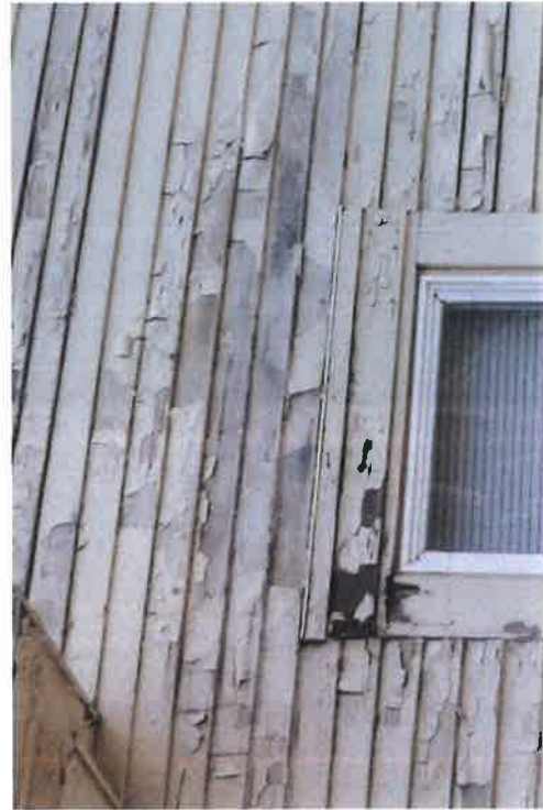
TYPICAL CLAPBOARD CONDITIONS SUMMER STREET BLOCK - BIDDEFORD, MAINE NOT FOR CONSTRUCTION (FOR HISTORIC APPLICATION ONLY)
