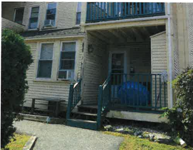
Existing Rear Porch
