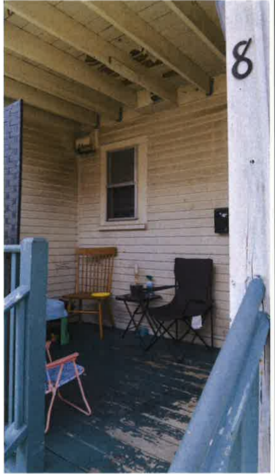
16 | Rear (North) Elevation - rear porch at #8
