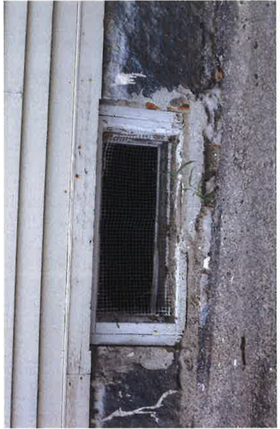
23 | East Elevation - basement window
