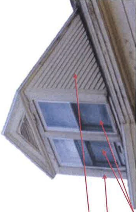
TYPICAL DORMER AT REAR (WINDOWS REPLACED)
