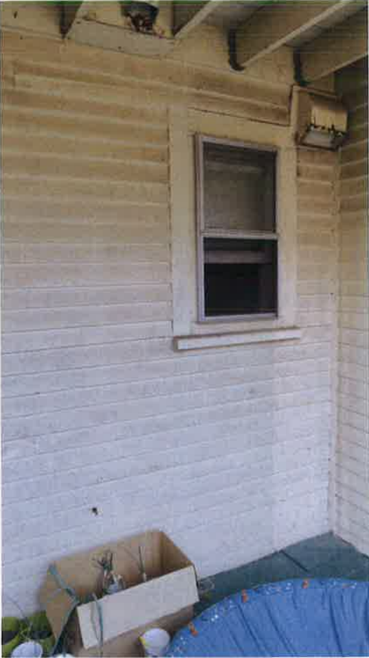
18 | Rear (North) Elevation - typical original window at rear
