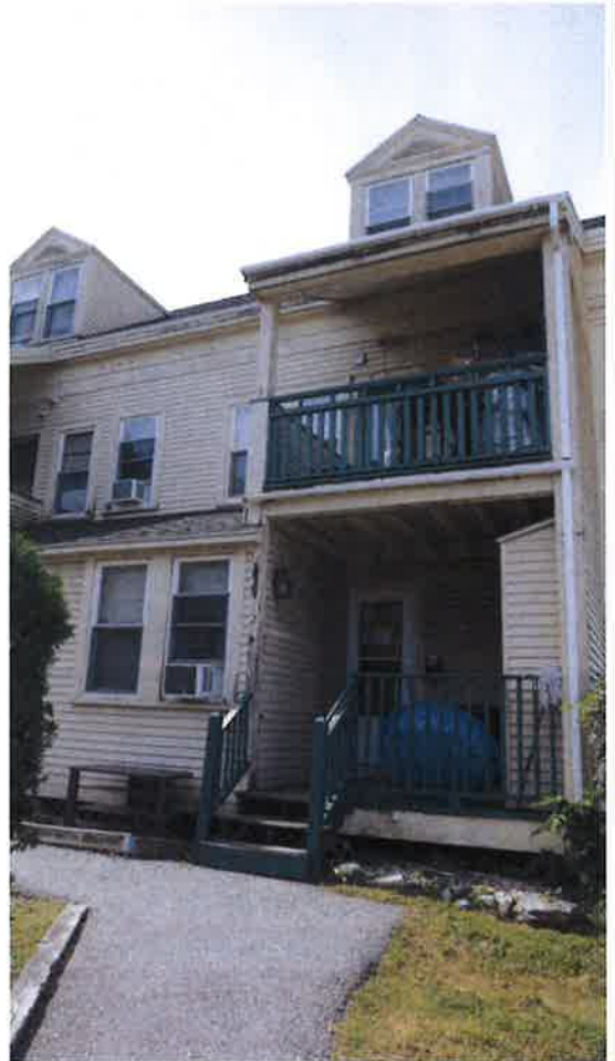
15 | Rear (North) Elevation - detail at west end
