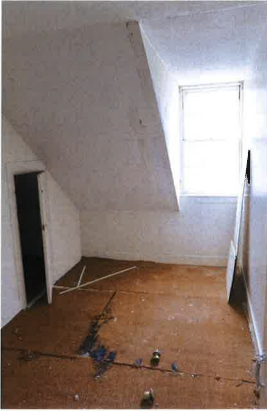
29 | 1 Summer Street - third floor - southeast bedroom
