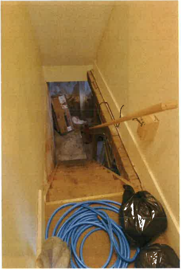
44 | 6 Summer Street - first floor - stair to basement
