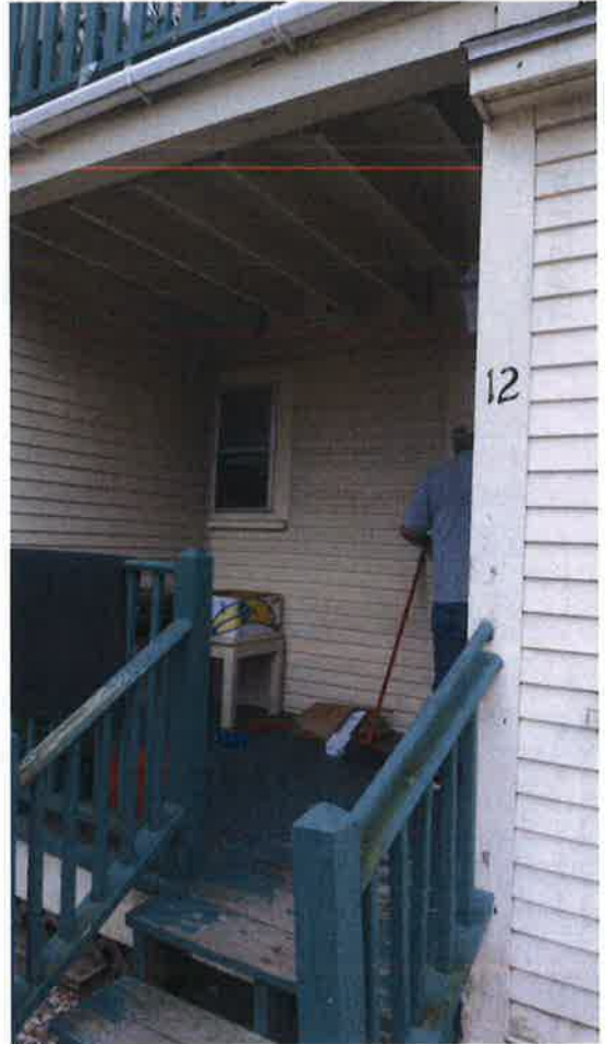
19 | Rear (North) Elevation - rear porch at #12
