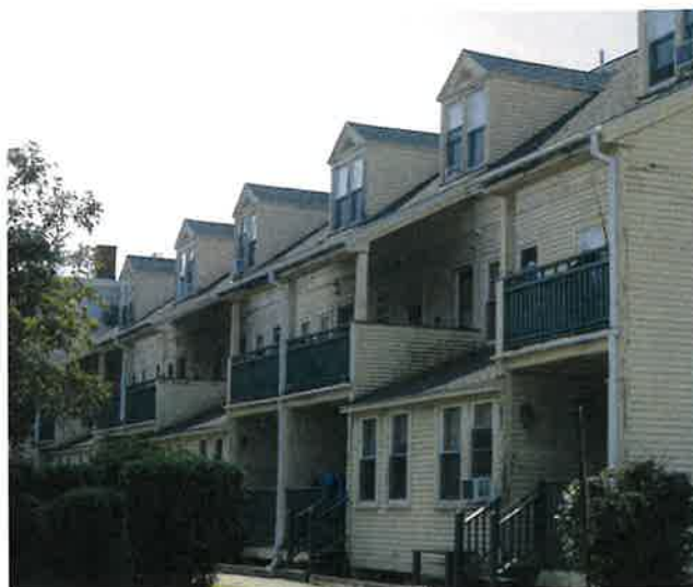
Existing Rear Porches
