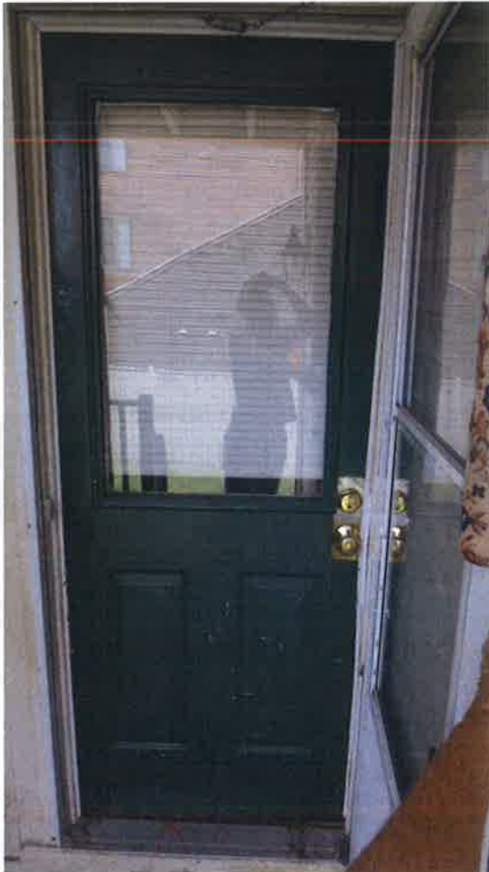
17 | Rear (North) Elevation - typical rear entrance
