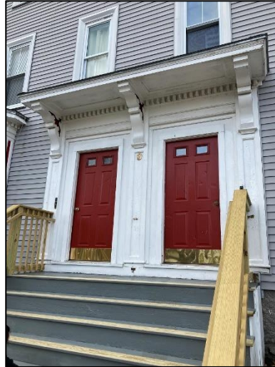
Right: Front Entry. Existing handrails will remain. Far right: Existing cellar windows at bays will be replaced.
