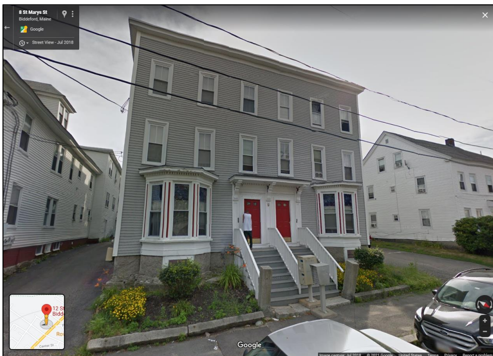
Source: "9 St. Mary's Street, Biddeford, Maine." 43°29'39" N 70°27'30" W. Google Earth Street View. Imagery Date: 07/2018. Accessed Date: 11/02/2021.
