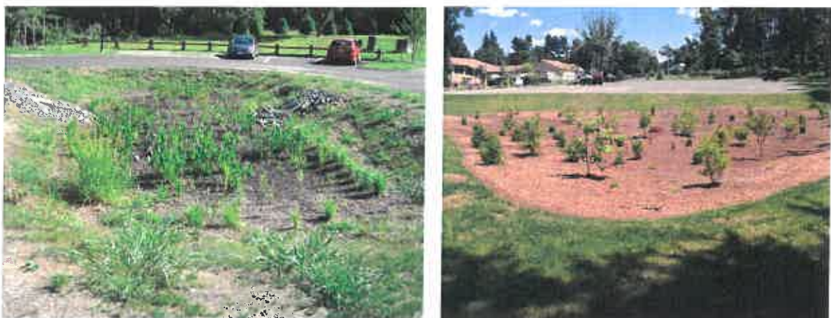
Example rain gardens after construction.
