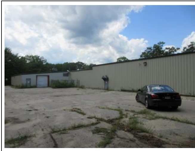
13) Easterly (rear) building elevations
