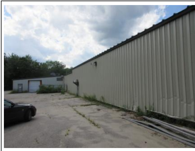
14) Easterly building elevation
