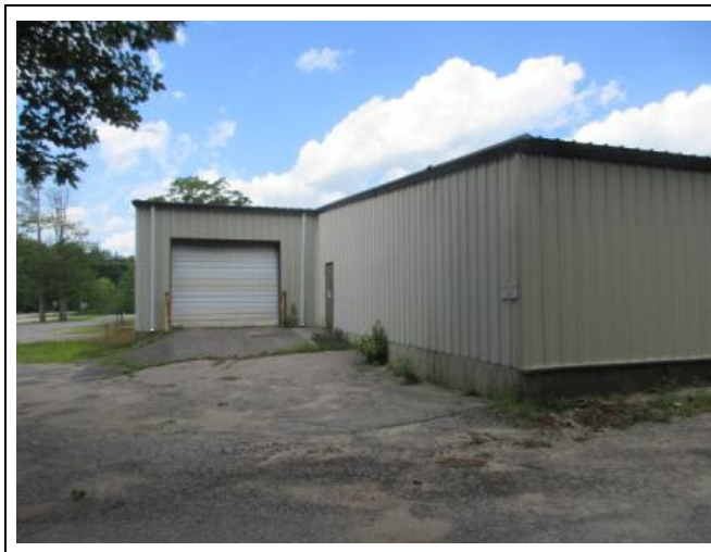
11) Southerly building elevation
