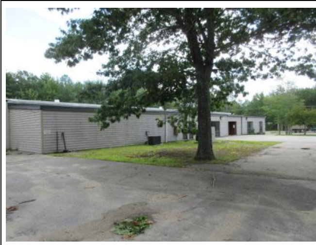
3) Westerly elevation of office section
