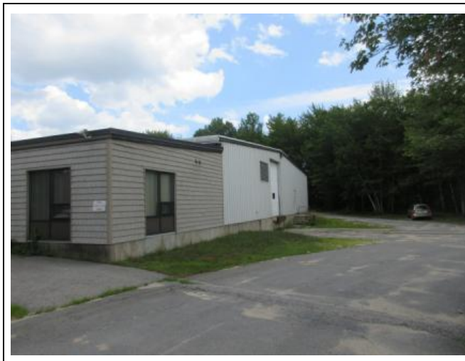
7) Southerly building elevation
