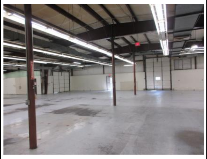
32) Original production floor looking toward loading door
