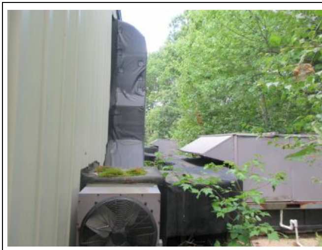
15) Northerly elevation showing exterior air handlers
