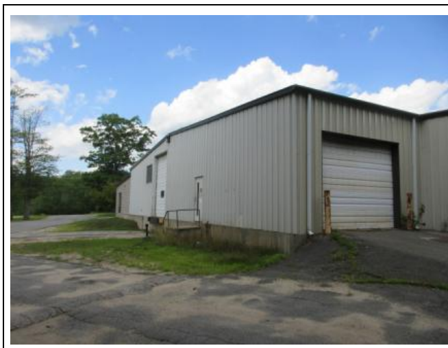
9) Southerly building elevation
