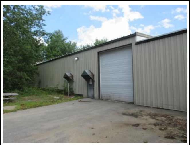
4) Westerly elevation of newer production addition
