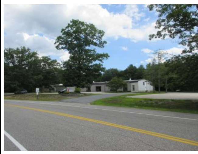
1) Westerly (front) and southerly building elevations
