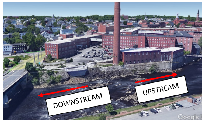
View of site prior to wall failure (googlemaps.com)
