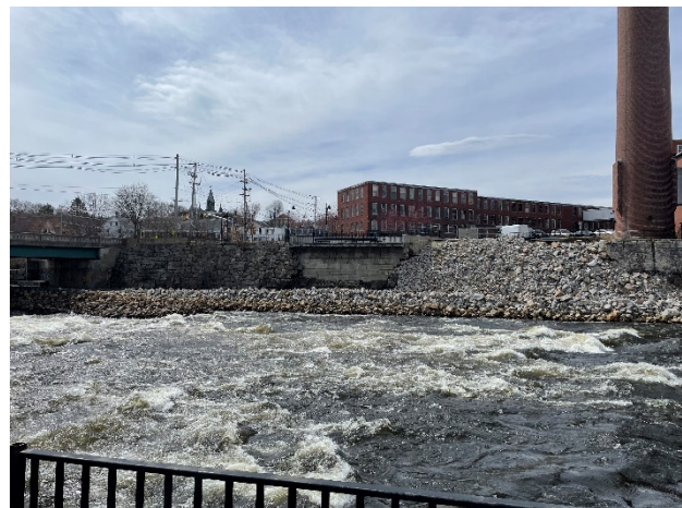
Emergency Repair Measure
