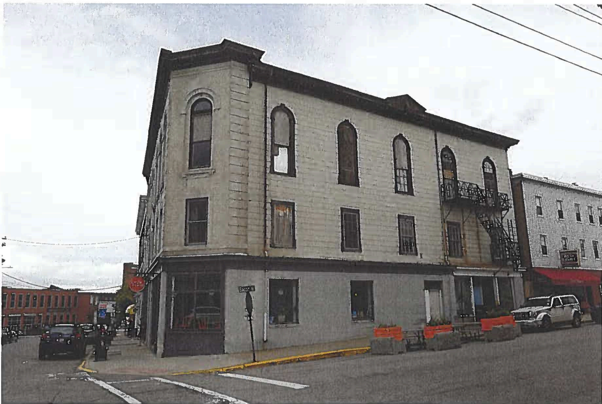
Photograph 4. The south or Bacon Street facade. International Order of Odd Fellows (IOOF) Building, 25 Alfred Street, Biddeford, ME. July 1, 2021.
