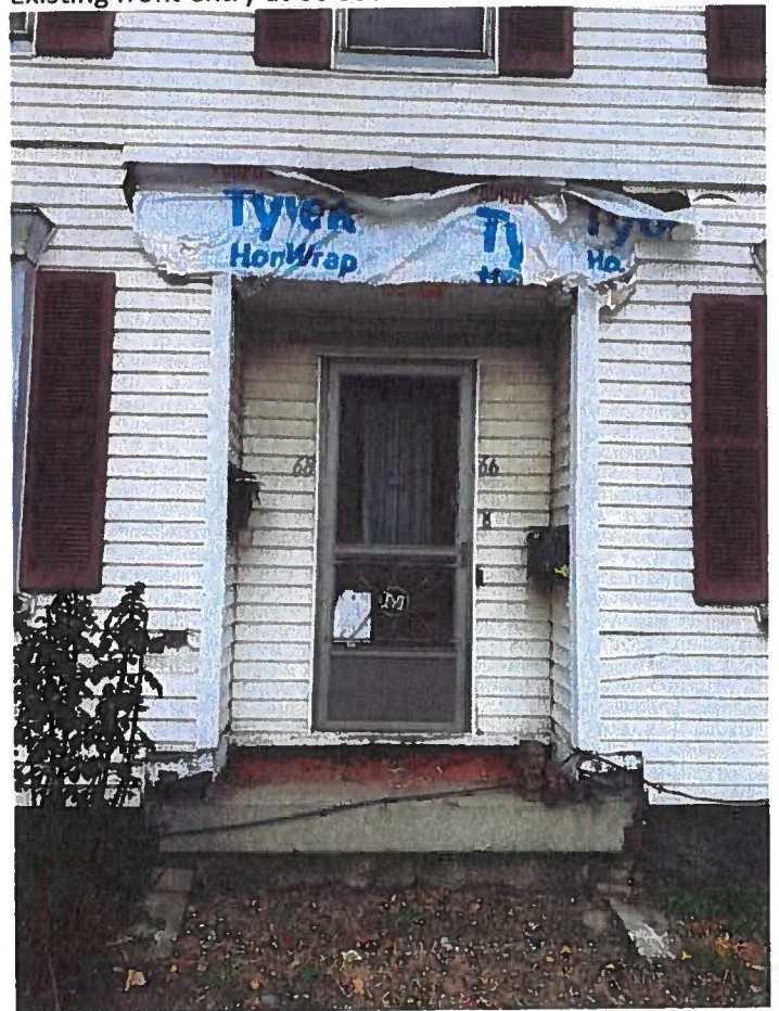
Existing front entry at 66 South
