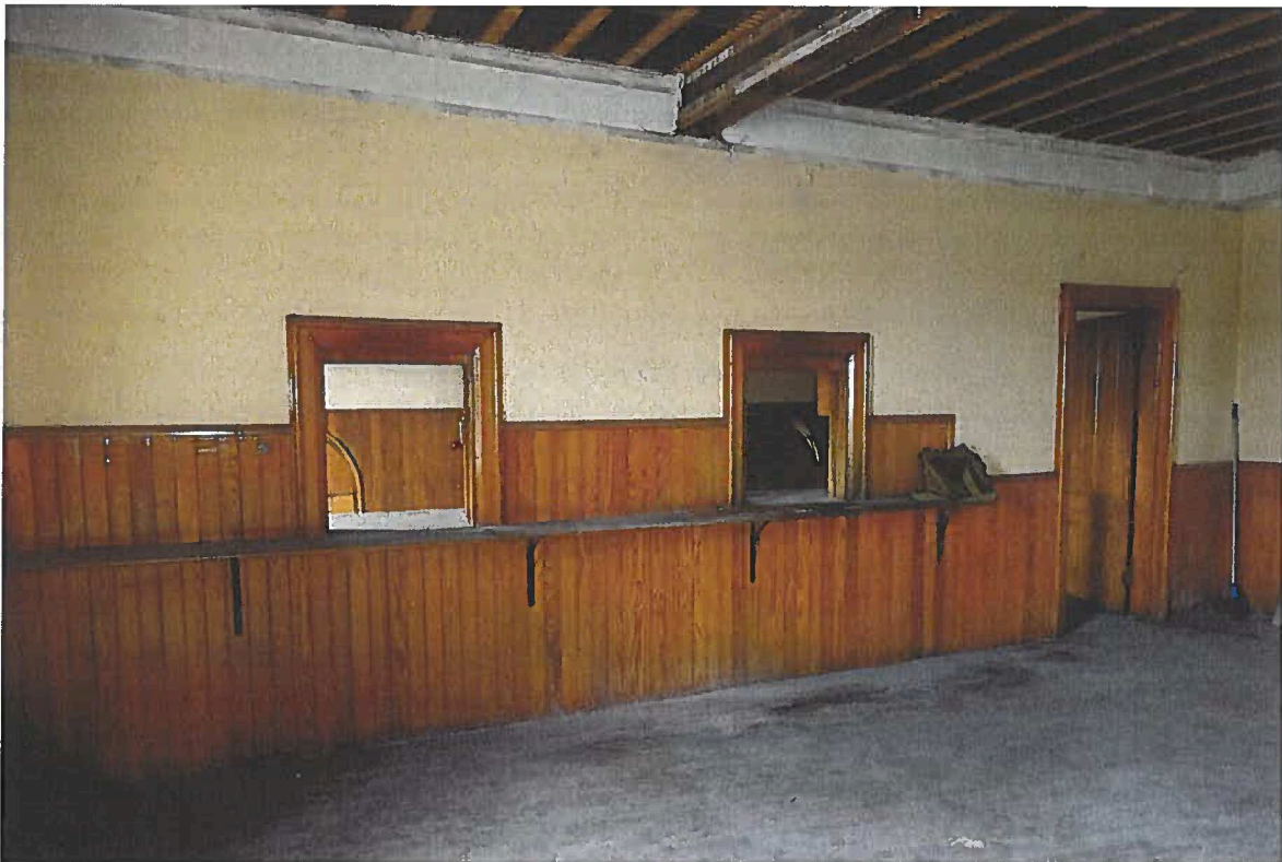
Photograph 20. International Order of Odd Fellows (IOOF) Building, 25 Alfred Street, Biddeford, ME. July 1, 2021.
