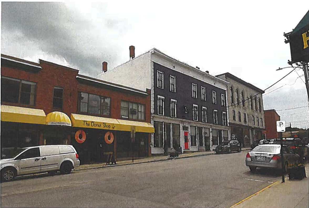
Photograph 2. Context shot, looking southwest down Alfred Street. International Order of Odd Fellows (IOOF) Building, 25 Alfred Street, Biddeford, ME. July 1, 2021.
