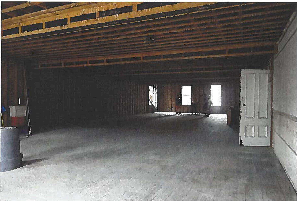
Photograph 10. International Order of Odd Fellows (IOOF) Building, 25 Alfred Street, Biddeford, ME. July 1, 2021.
