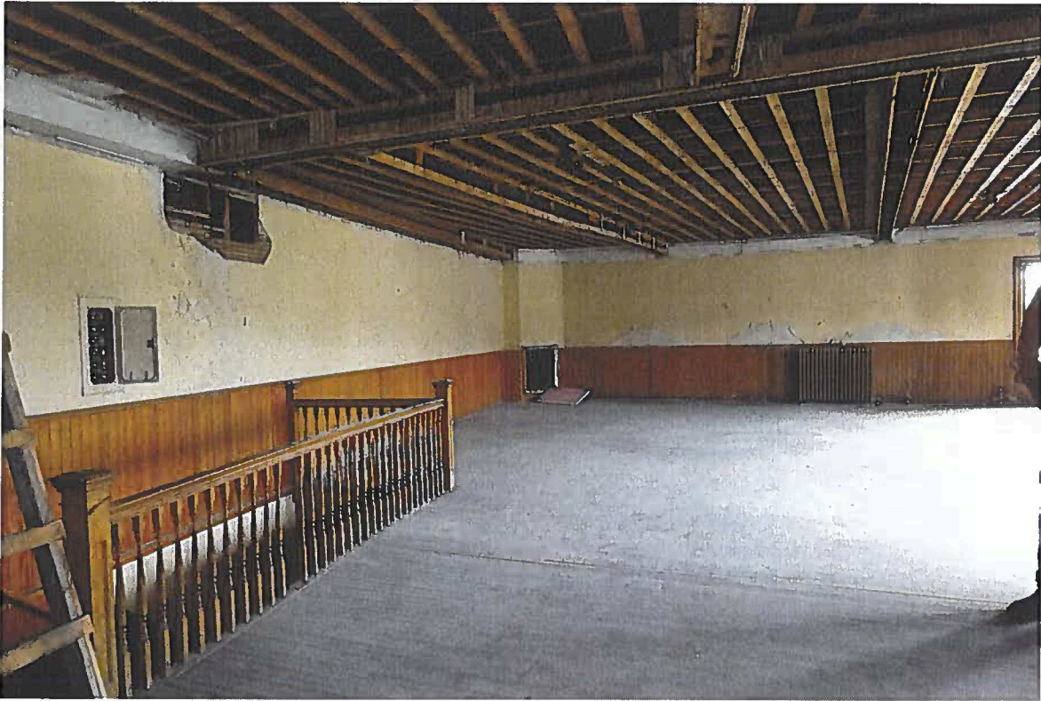
Photograph 19. International Order of Odd Fellows (IOOF) Building, 25 Alfred Street, Biddeford, ME. July 1, 2021.
