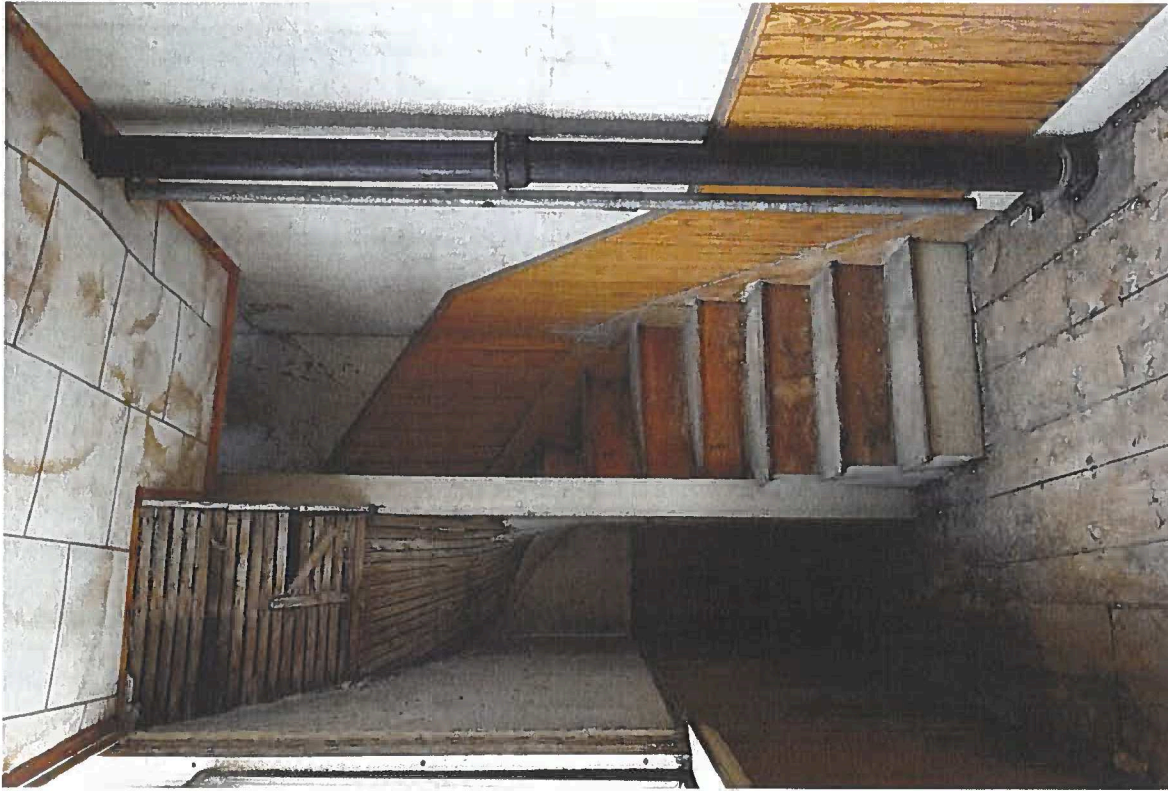
Photograph 21. Stairs to loft. International Order of Odd Fellows (IOOF) Building, 25 Alfred Street, Biddeford, ME. July 1, 2021.
