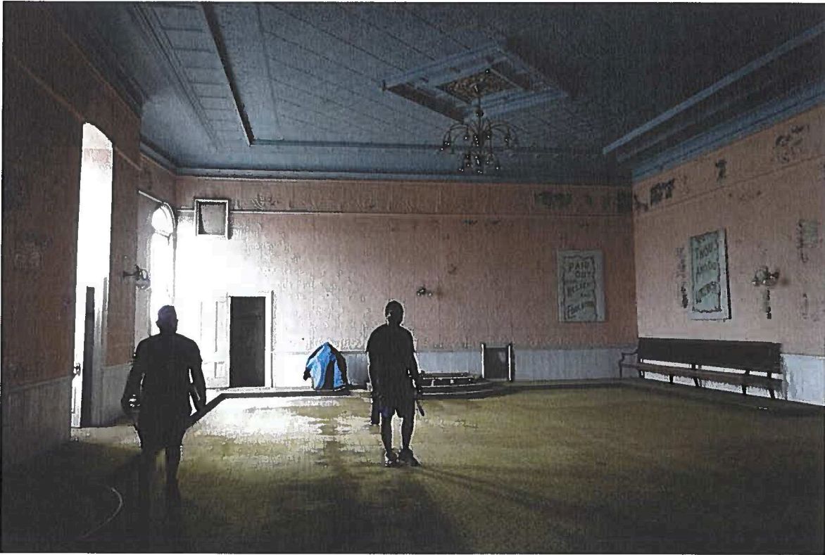
Photograph 17. International Order of Odd Fellows (IOOF) Building, 25 Alfred Street, Biddeford, ME. July 1, 2021.
