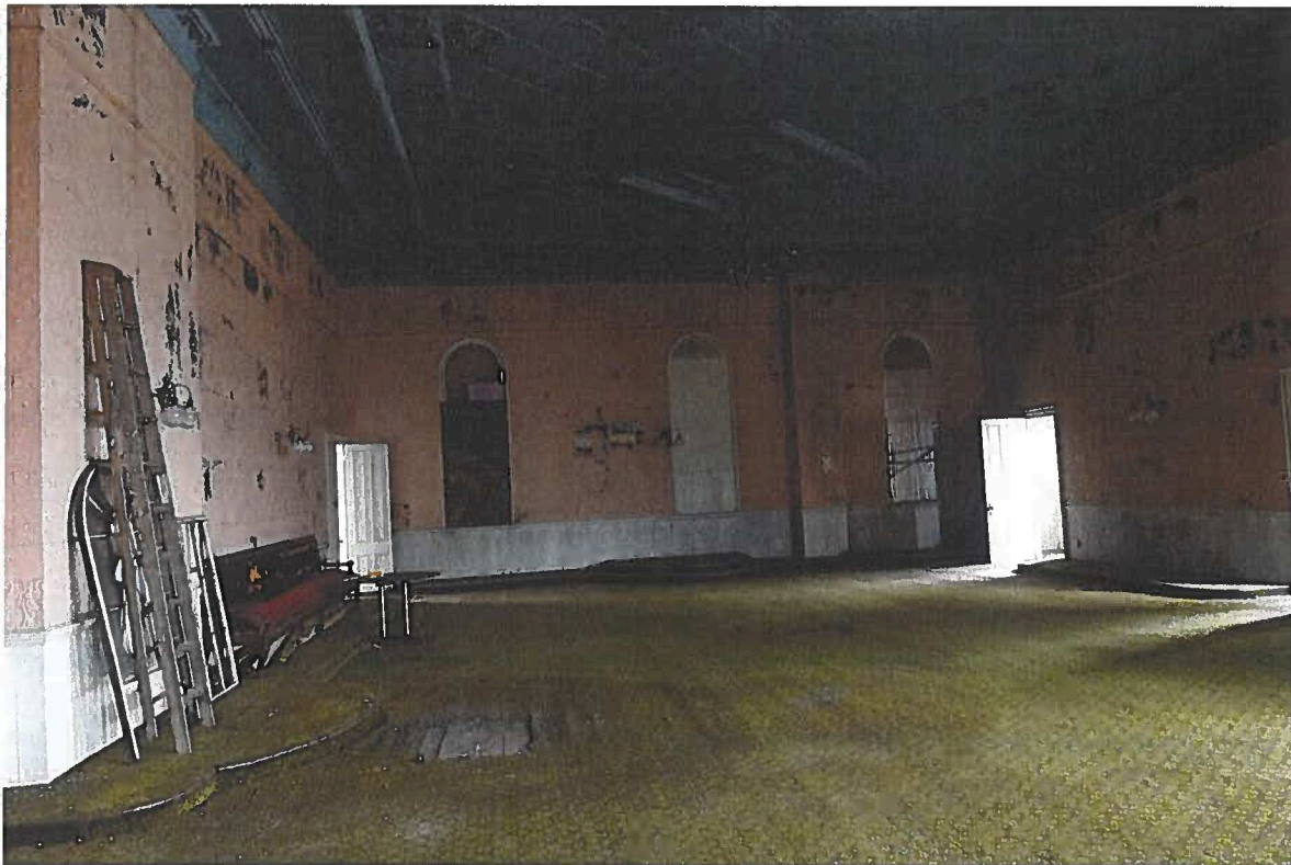
Photograph 16. International Order of Odd Fellows (IOOF) Building, 25 Alfred Street, Biddeford, ME. July 1, 2021.
