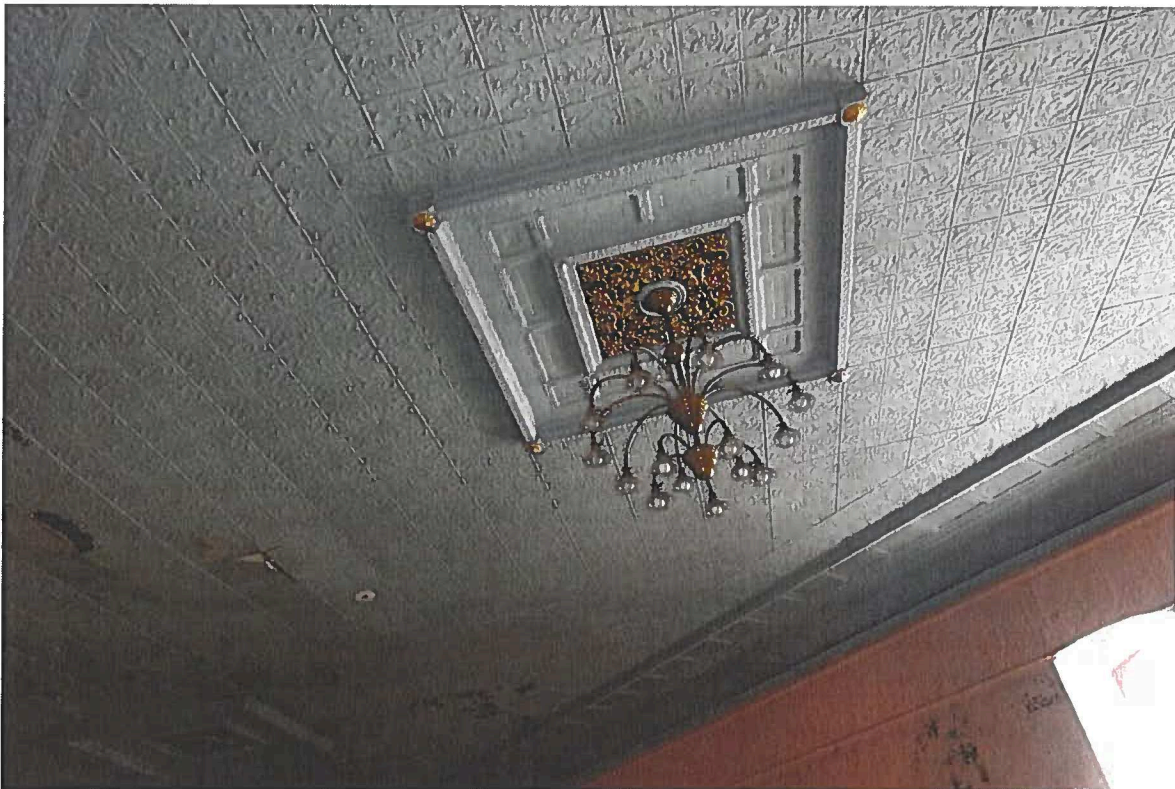
Photograph 18. International Order of Odd Fellows (IOOF) Building, 25 Alfred Street, Biddeford, ME. July 1, 2021.
