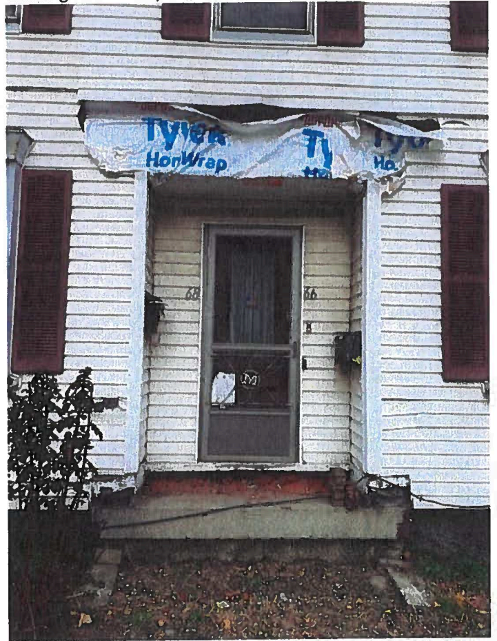
Existing front entry at 66 South
