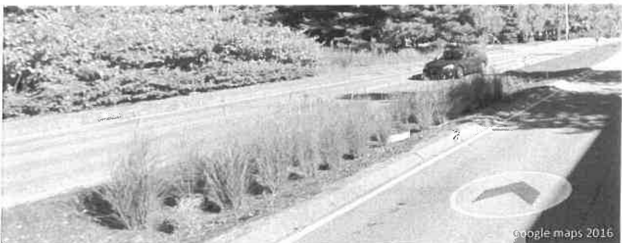
Linear gravel wetland, Gorham Road, South Portland, ME
