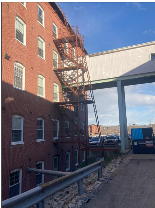
The view from the southwest corner of the building.
