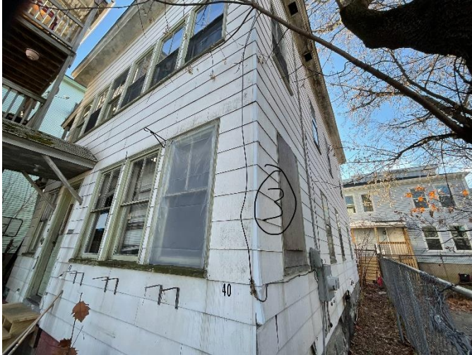
Right side - One window will be replaced here.
