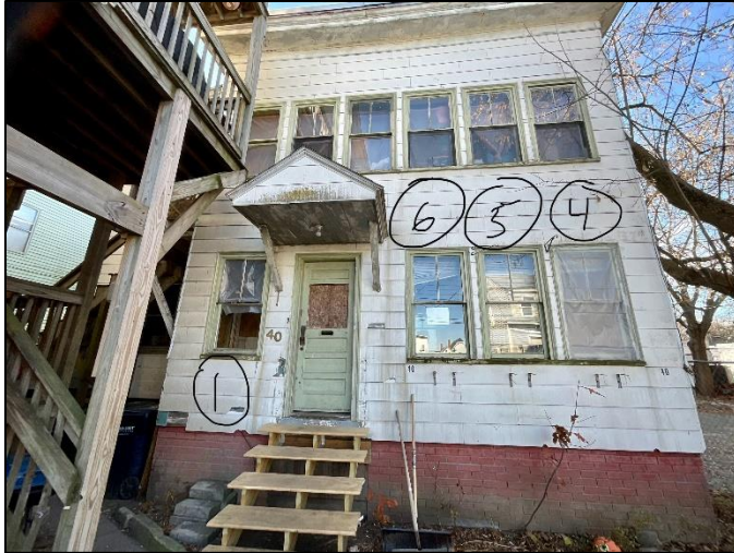
Front - Four Windows will be replaced here.
