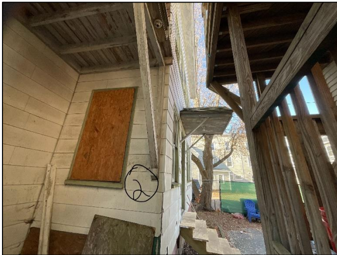
Left side - One window to be replaced here.
