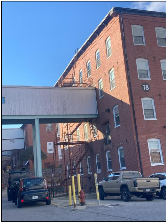
From the parking lot, the fire escape is partially obscured by the enclosed bridge to Building 19.
