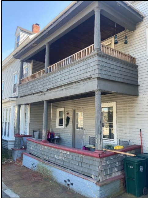
Existing overall conditions.
