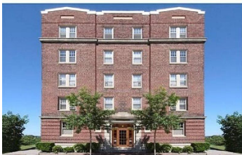
11 Shepley – 40 Unit Market Rate Apartment Building in Portland, Maine, pre-negotiated master lease with Maine College of Art – Sold as part of a 1031 Exchange
