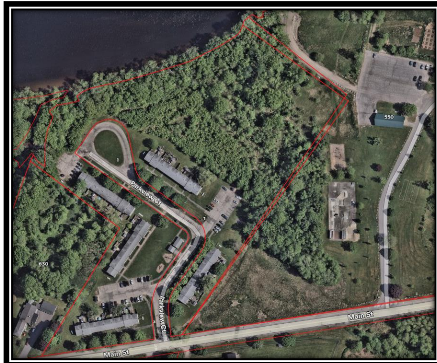
Forest Green Apartments – Existing Conditions
