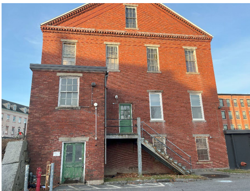
Figure 2: View of the east side of Building 30 facing west.
