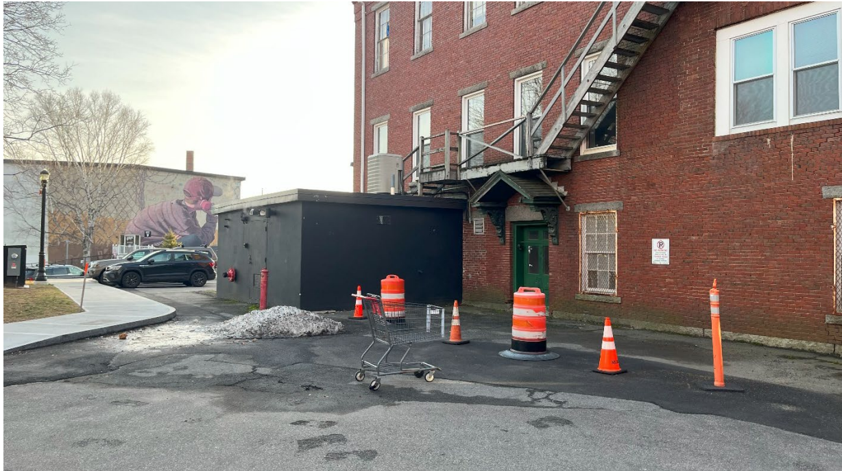
Figure 5: Overview of north side of building.
