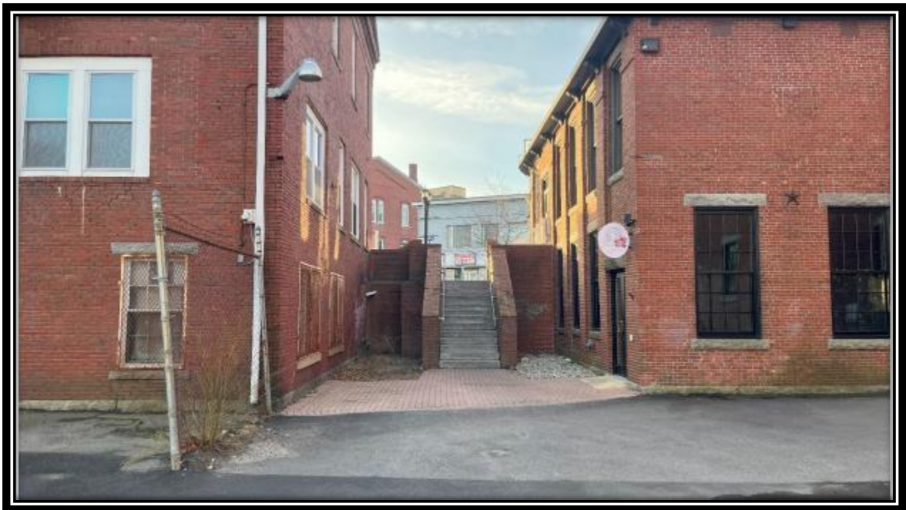
Pepperill Mill - Building # 30 – 2 York Street – Rear Façade (left) – Stairs to Main Street
