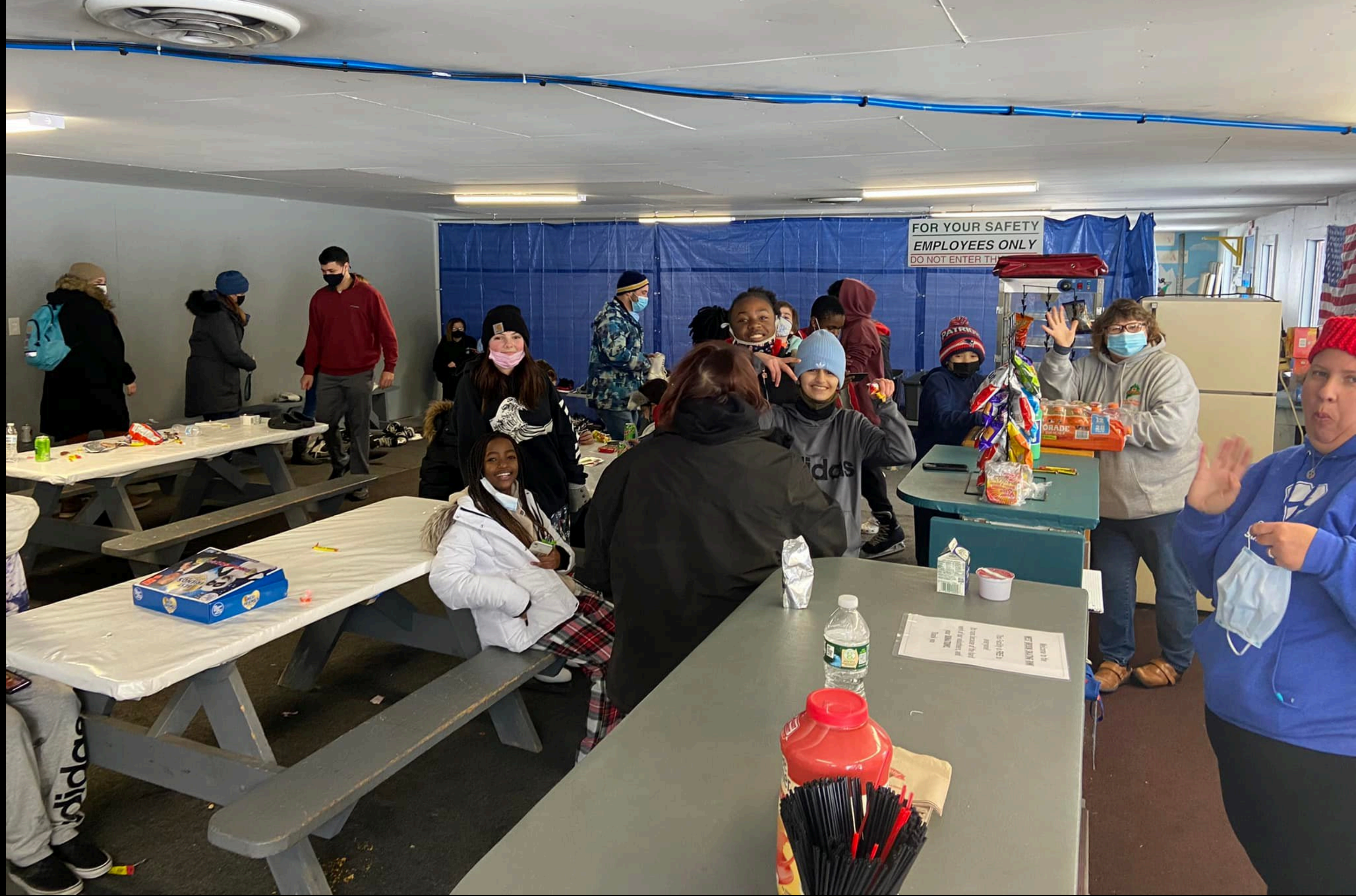
With the floor having major issues only 1/3 of the building was used.
