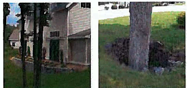
The retaining wall (l) was used to minimize grading that could have harmed the adjacent trees. The tree well (r) should have extended out to the drip line to protect the root system near the surface.
