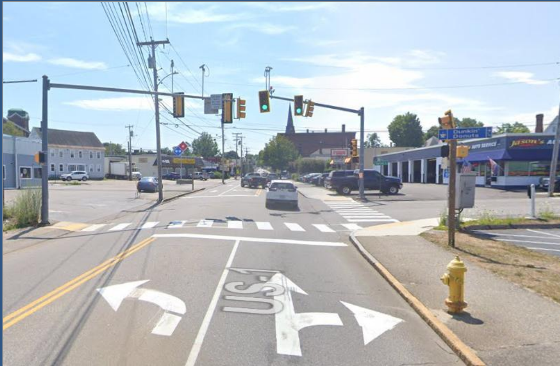
Existing Spruce St. signalized intersection looking SW on Elm St.
